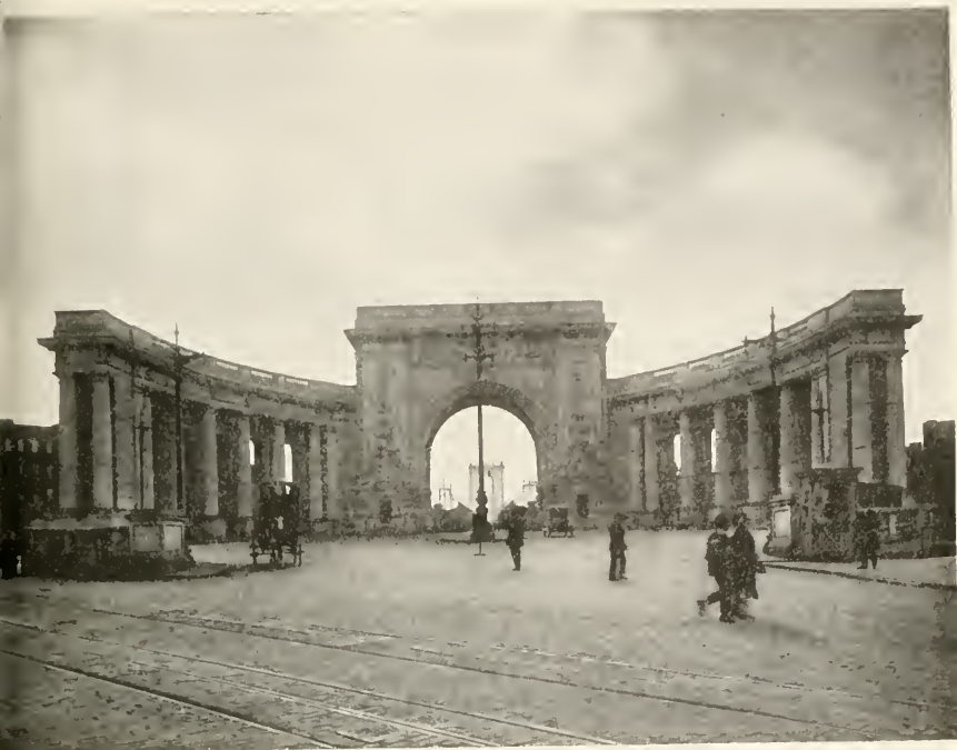
MANHATTAN BRIDGE, BOWERY TERMINAL CARRÈRE AND HASTINGS, ARCHITECTS SCULPTURE BY RUMSEY AND HEBER (PAGE 177)
