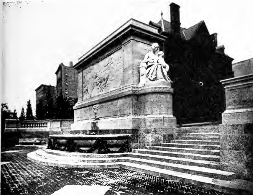
FIREMEN'S MONUMENT, RIVERSIDE DRIVE H. VAN BUREN MAGONIGLE, ARCHITECT ATTILIO PICCIRILLI, SCULPTOR (PAGE 350)
