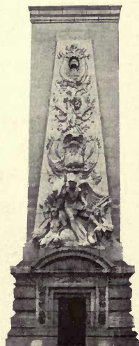
DECORATIVE PANELS "COMMERCE" CARL A. HEBER, SCULPTOR DETAIL MANHATTAN BRIDGE BOWERY TERMINAL
