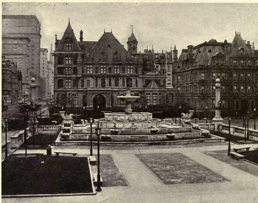
THE PLAZA, LOOKING SOUTH, SHOWING THE FOUNTAIN OF ABUNDANCE AGAINST THE CORNELIUS VANDERBILT HOUSE CARRÈRE AND HASTINGS, ARCHITECTS (PAGE 308)
