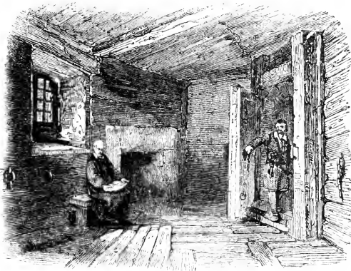
INTERIOR OF LOLLARDS TOWER
