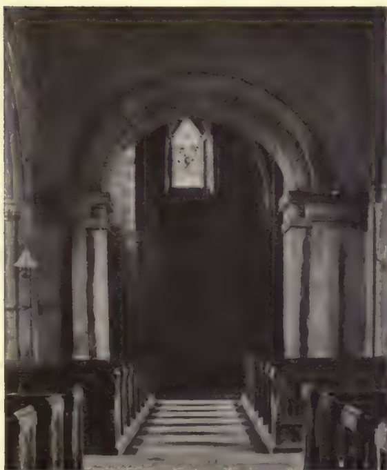
Fig. 597.—Barnack Church. Tower arch (XIth Century).
