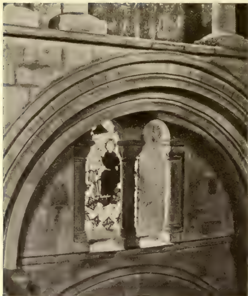
Fig. 670.—Oxford Cathedral. Opening in quasi-triforium (XIIth Century).
