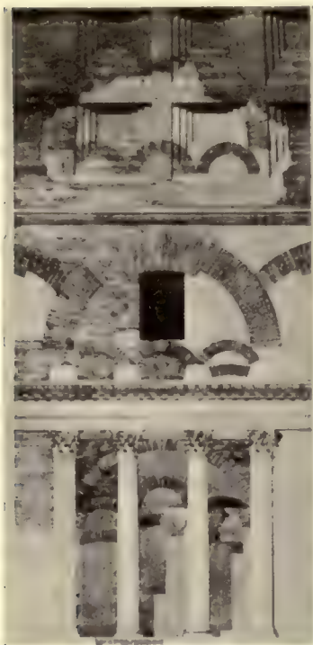
Fig. 486.—Rome. Pantheon. System of relieving arches (120-124). (From Beltrami, "Il Pantheon.")
