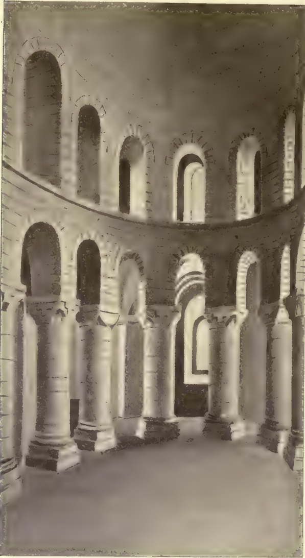
Fig. 637.—Tower of London. St. John's Chapel (about 1080). (From a sketch by Miss P. Bruce.)
