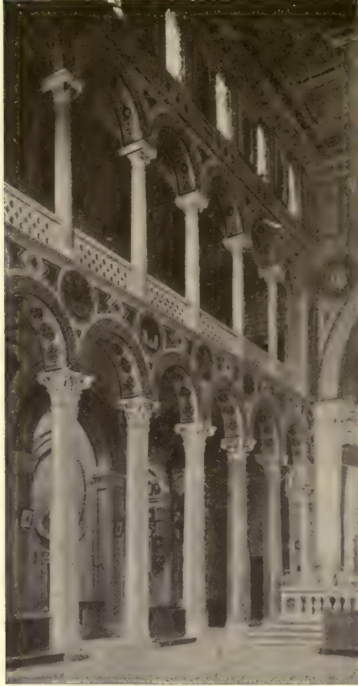
Fig. 532.—Rome. Basilica of Sant' Agnese outside the walls (VIIth Century).
