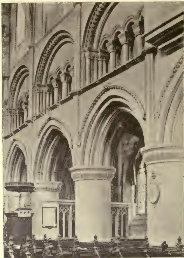
Fig. 682.—Malmesbury Abbey Church. Nave (XIIth Century).
