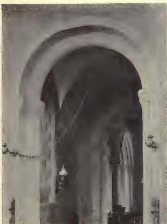
Fig. 615.—Langford Church. Tower arches (XIth Century).
