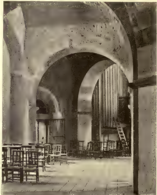
Fig. 719.—Aachen. Palace Chapel. Vaulting in the gallery (796–804).
