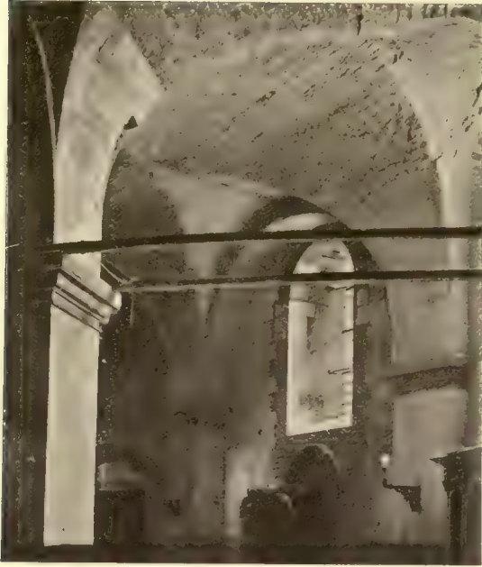
Fig. 718.—Aachen. Palace Chapel. Vaulting of aisle (796–804).
