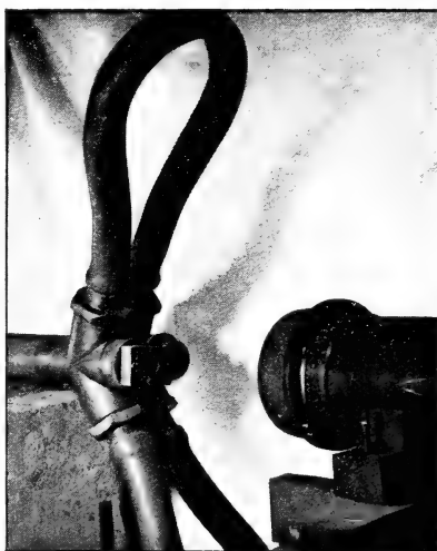
FIG. 6.—Showing further end of pipe-line.
