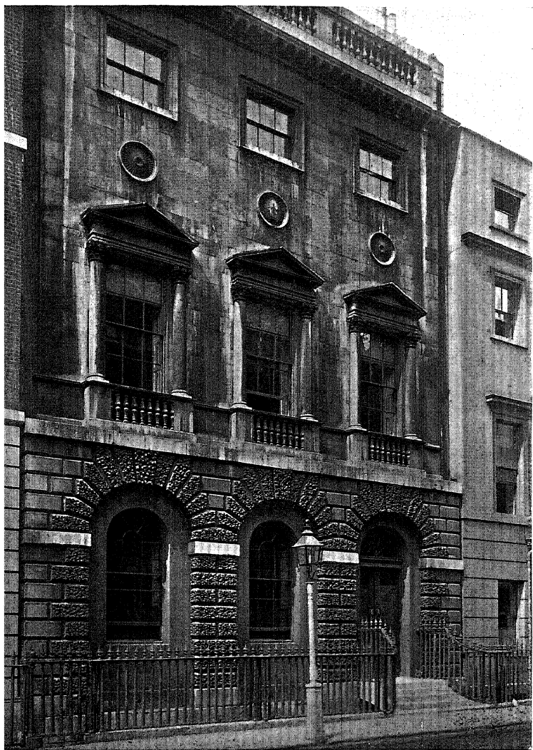
Ely House, Dover Street, Designed by Sir Robert Taylor for Bishop Keen in 1772.
