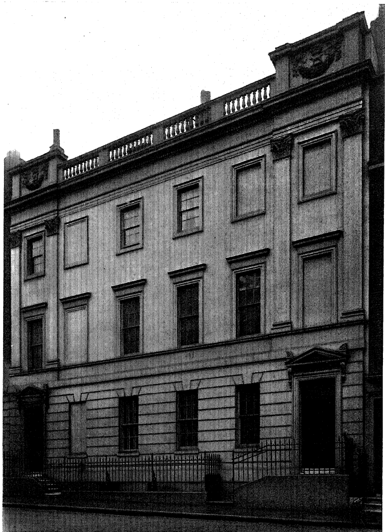
The Westminster Estate Office, No. 53 Davies Street, W. (1820).
