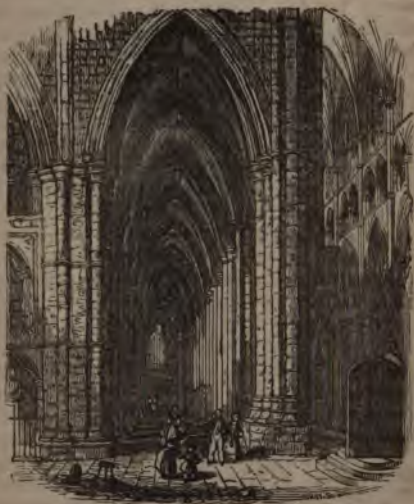
SOUTH AISLE OF THE NAVE.
