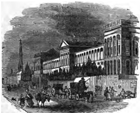
ST. LUKE'S HOSPITAL.
