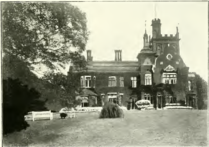
CAEN WOOD TOWERS (South View)
