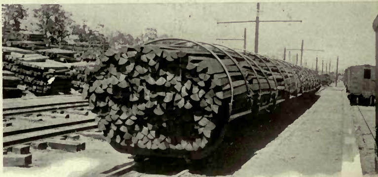
This picture shows a charge of posts (16 cages or tram cars) after leaving treating plant. Note creosoted ties in background.
