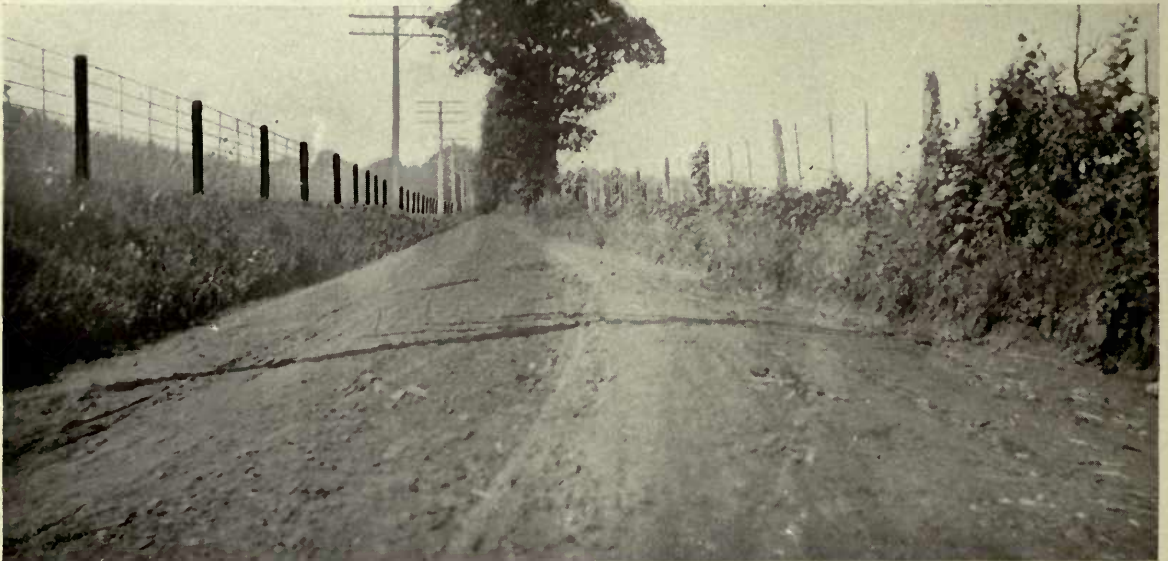
The old and the new. On the left is seen fence strung on Long-Bell Creosoted Yellow Pine Posts—good for fifty years. On the right, a makeshift fence—home-made posts, untreated, with steel rods in between.
