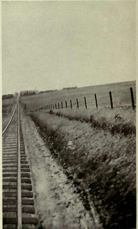
In the interest of neatness, economy and safety, many railroads have adopted creosoted posts for right-of-way fencing. They are fire-resistant.
