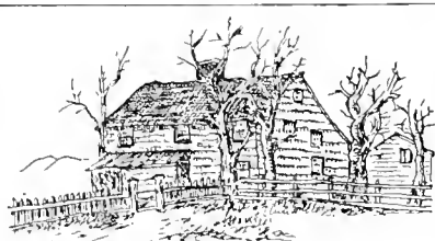
SAYRE HOUSE, SOUTHAMPTON. Recently Condemned.
