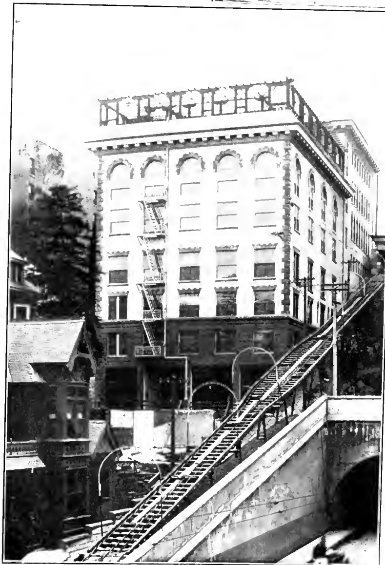
LOOKING FROM HILL STREET
