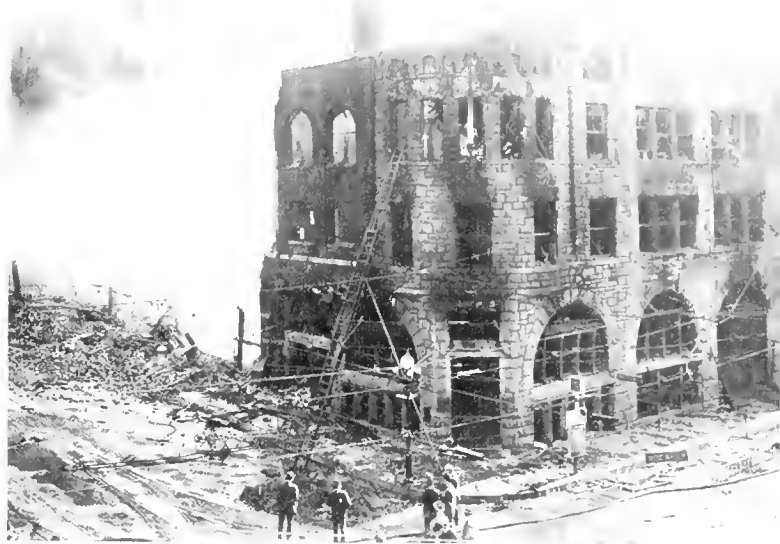
Times building following bombing in 1910. Reports following explosion stated that the amount of dynamite would not have caused such extensive damage; gas leakage in the plant created a greater explosion.
