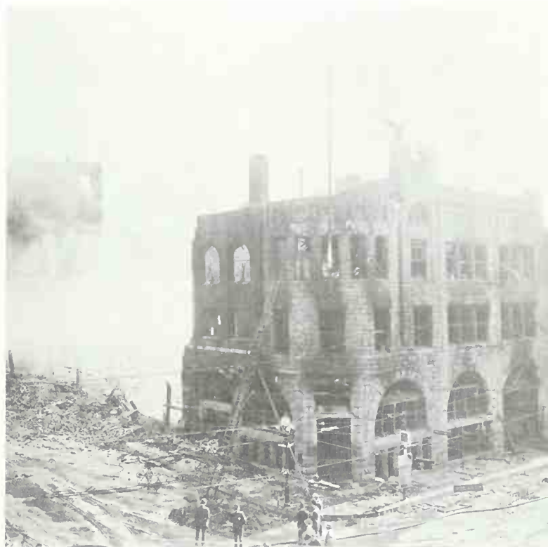
Times building following bombing in 1910. Reports following explosion stated that the amount of dynamite would not have caused such extensive damage; gas leakage in the plant created a greater explosion.
