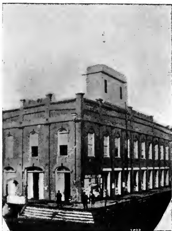
OLD COURT HOUSE
