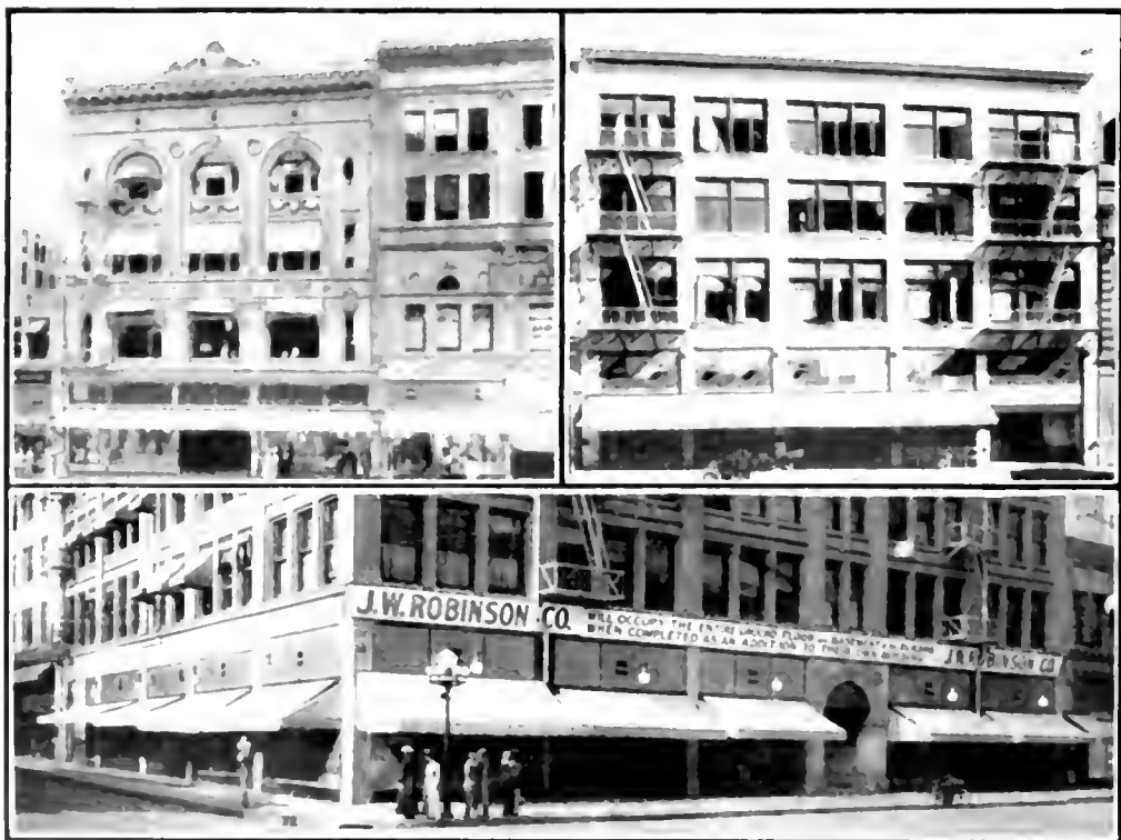
ADDITION, E. J. BYRNE BUILDING, THIRD STREET AND BROADWAY
