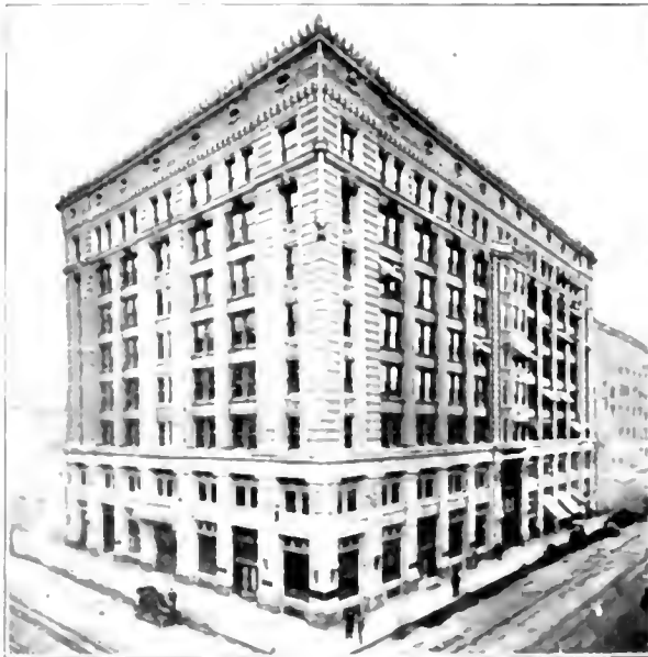
Third Home Security Savings Bank Spring and 4th Sts.
