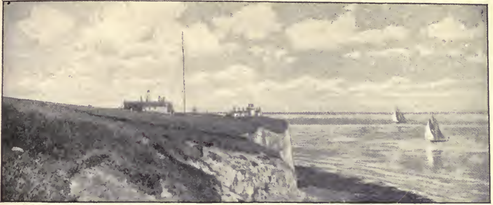
Experimental Station at South Foreland, showing the high pole, which is an essential feature of the Marconi system.
