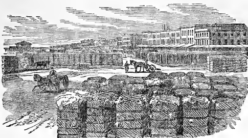
THE LEVEE AT NEW ORLEANS.
