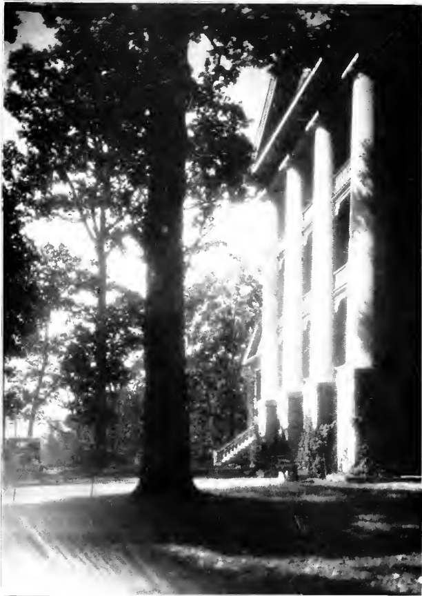
MAIN BUILDING (SIDE VIEW)
