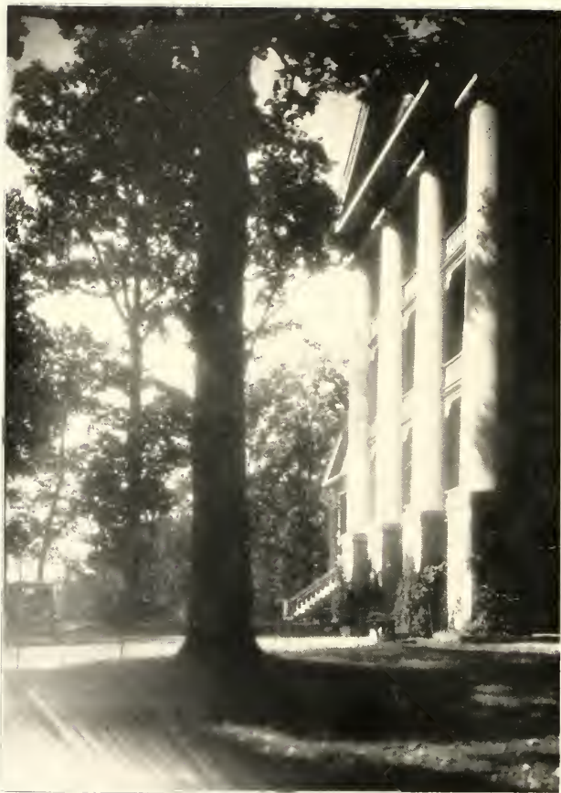
MAIN BUILDING (SIDE VIEW)
