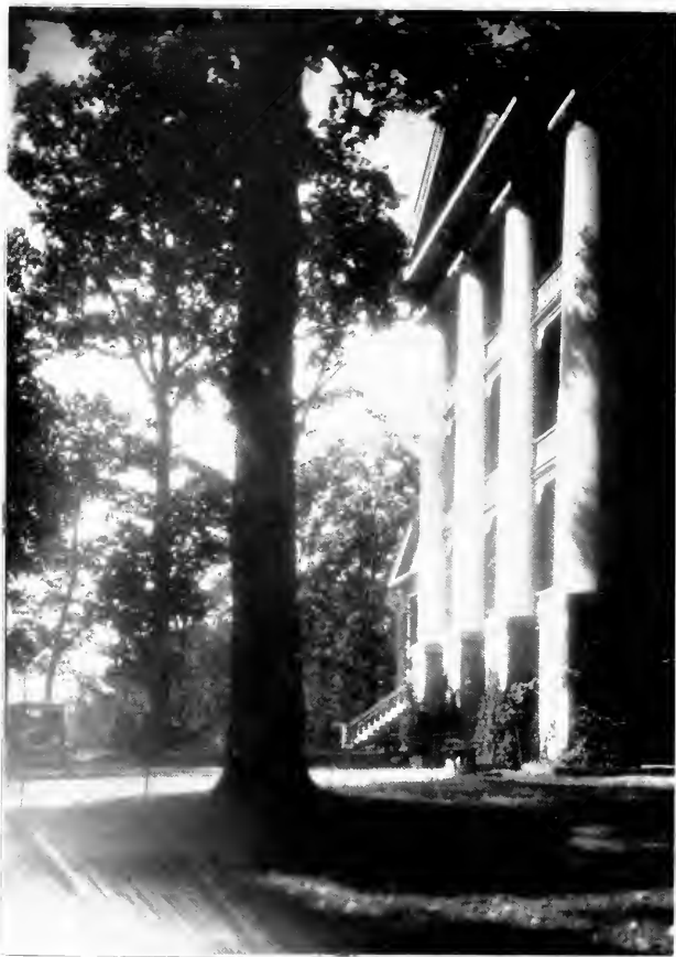
MAIN BUILDING (SIDE VIEW)
