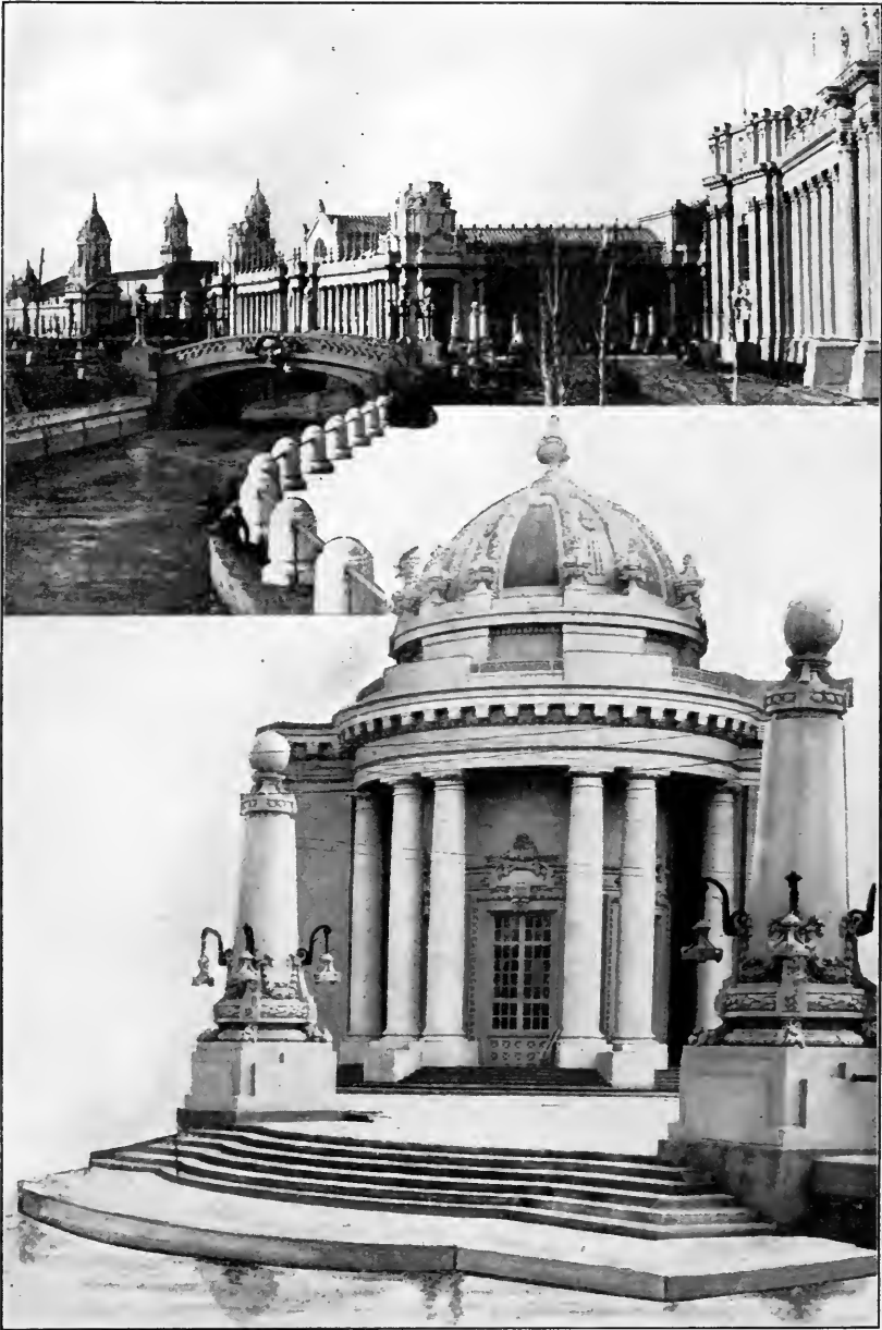
1. THE LAGOON, EAST OF MACHINERY HALL. 2. A CORNER OF THE PALACE OF LIBERAL ARTS.
