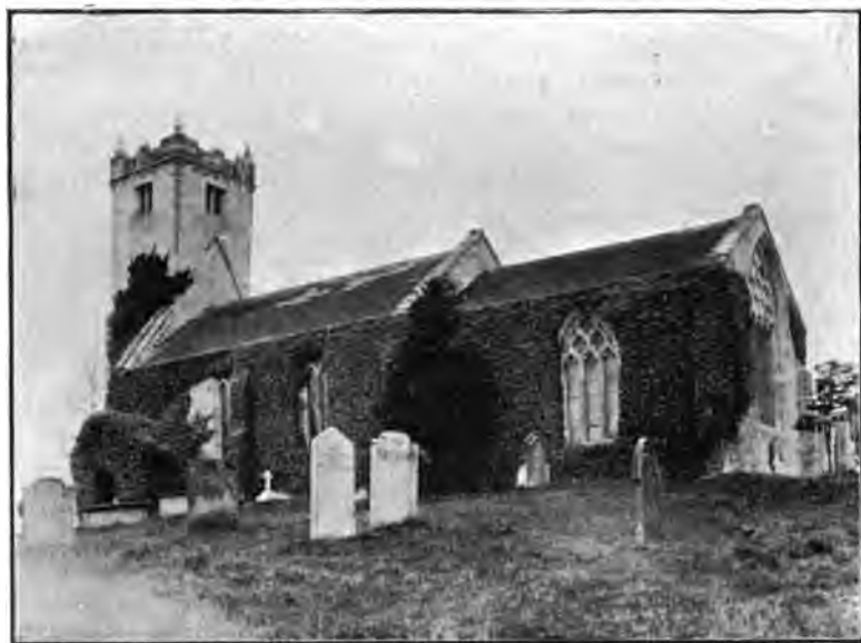
WALTON CHURCH BEFORE THE RESTORATION.
