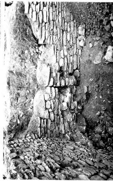
NORTH WALL, ROOM 18 (KIVA D), LOWRY PUEBLO; SHOWING METHOD OF ENLARGING ROOM BY EXTENDING WALL Gap between new and old walls (center) was only fortuitously discovered, so cleverly was it chinked up with mud mortar and spalls
