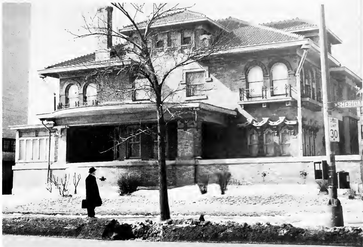
Rev. J. Donald Hayes, Director of Gonzaga Hall, gazes with satisfaction upon the new residence hall.
