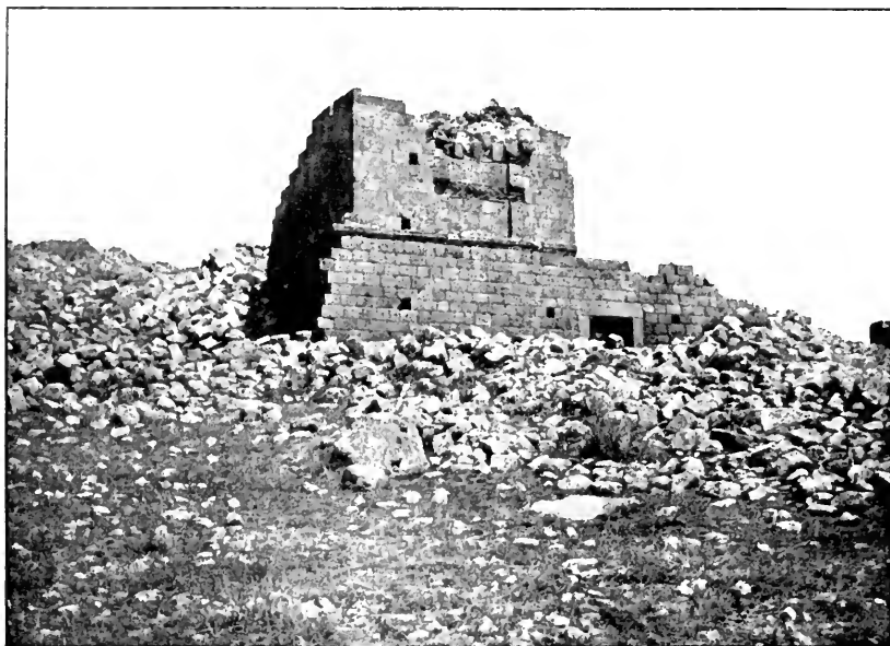
Part of a Monastery above Bin-Bir-Kilisse, showing short zones of brick used as ornament in a stone building.
