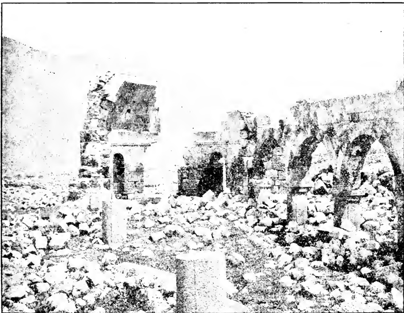
Church No. 5 at Bin-Bir-Kilisse, Apse and South Arcades of the Nave. To face p. 164. See pp. 155-161.
