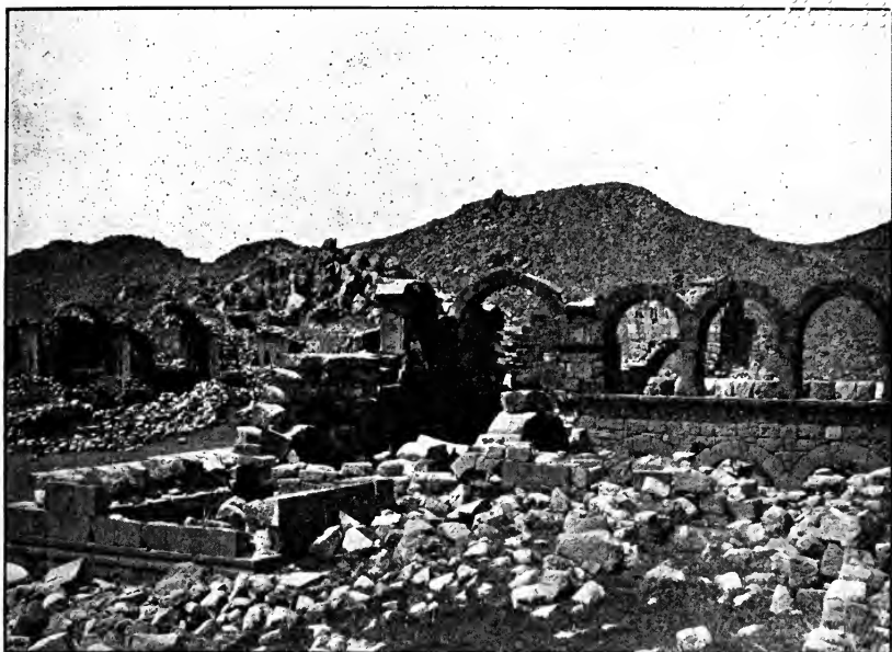
Church No. 32 at Deghile, looking from S.E. : North Arcades of the Nave : Chamber, South Extension of Narthex, on the left : Monastery Halls behind on left.
