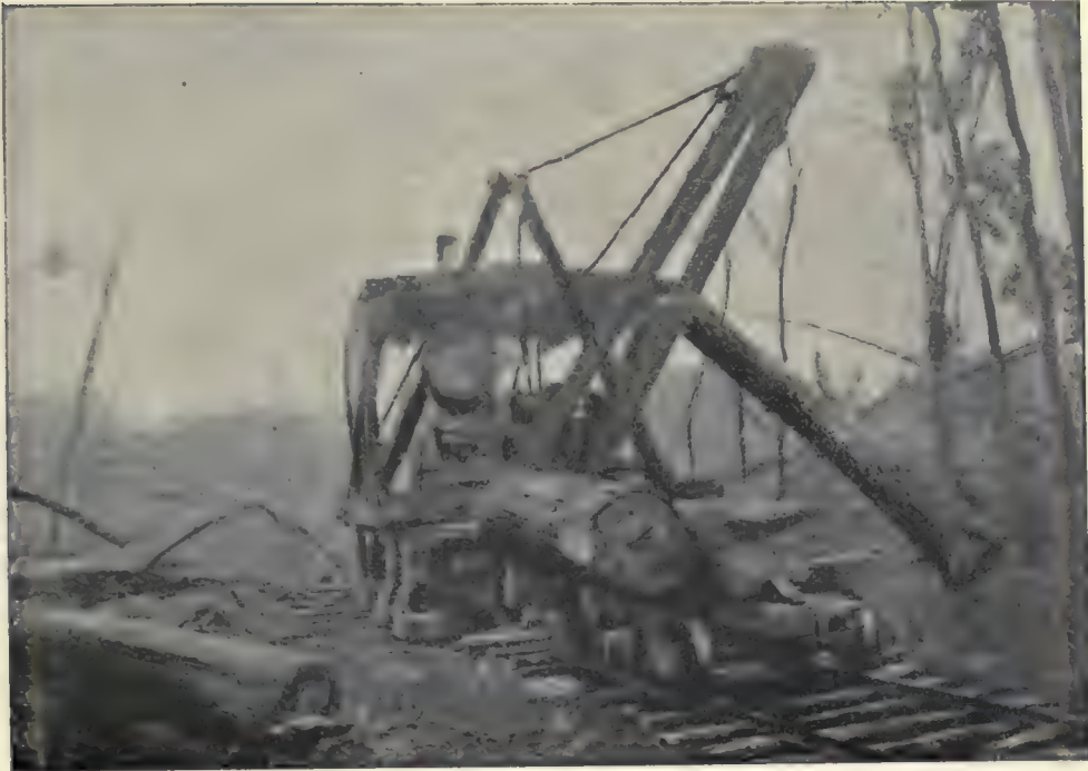
(1). Old Type of Lidgerwood Swinging Boom Loader mounted on a timber platform jacked up over the railway track.—Sardis, Mississippi.
