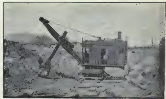
(3). Shovel mounted on railway track.
