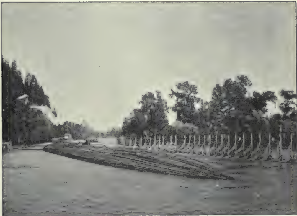
(2). Benson Raft completed ; cradle removed.
