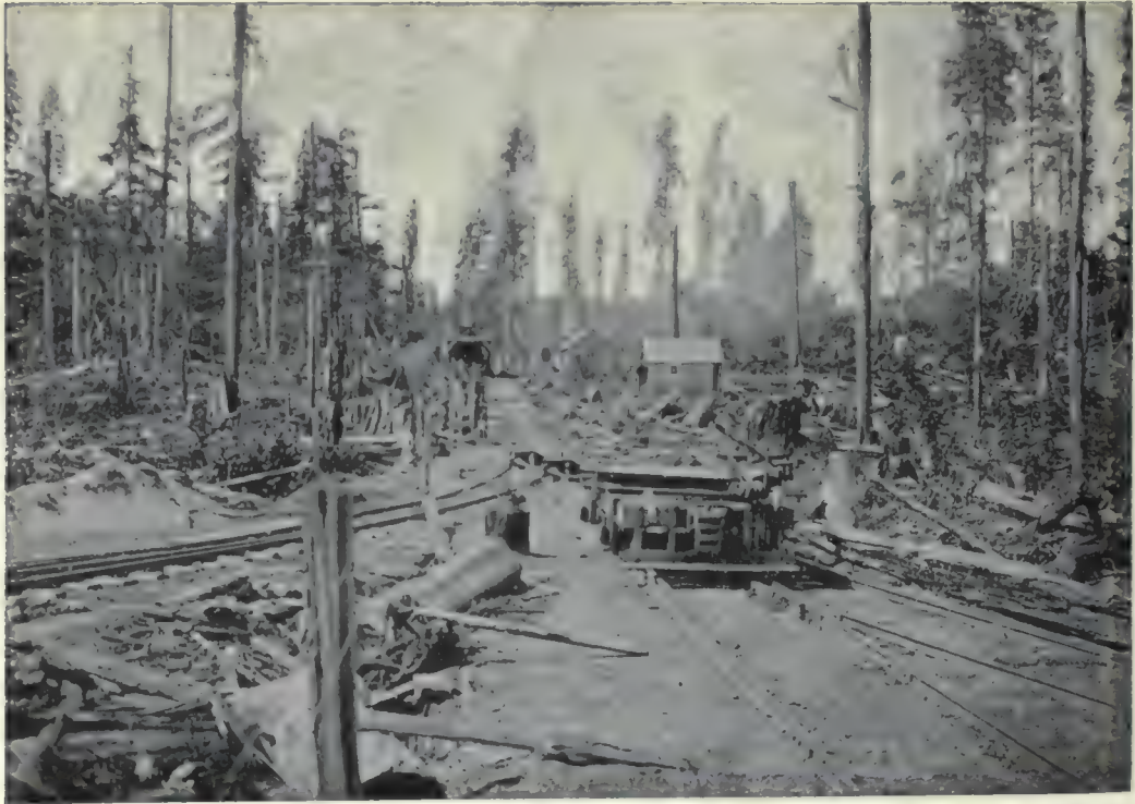
(1). Cable Railway or Incline ; special car for cable.—Arlington, Washington.
