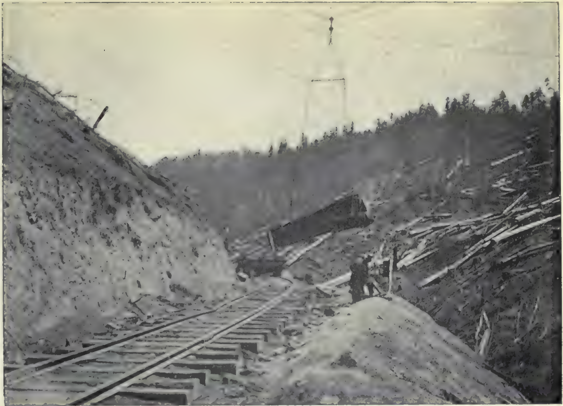
(1). SKY LINE SKIDDING AND LOADING. 8 ton log on 3 feet track ; telephone operator in the foreground.—Elk, California.
