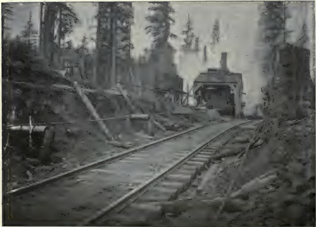
(2). Hoisting engine at top of Incline.—Arlington, Washington.
