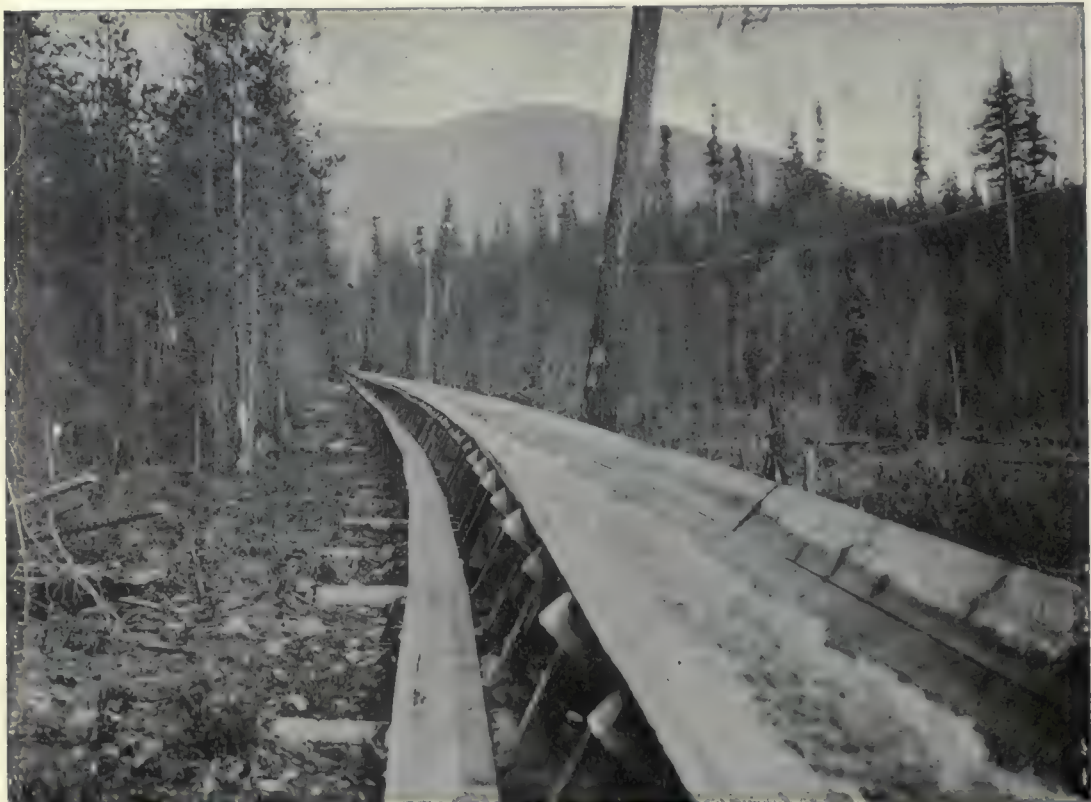
(2). Flume for logs up to 2 feet in diameter.—Addie, Idaho.
