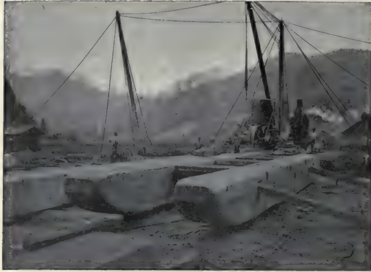
Timber skids for Skidder ; 40 feet \times 2 feet \times 2 feet Fort Bragg, California.
