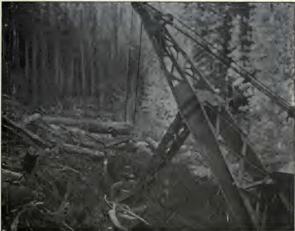
(2). Track being cleared by Shovel.—Elk River, Idaho.
