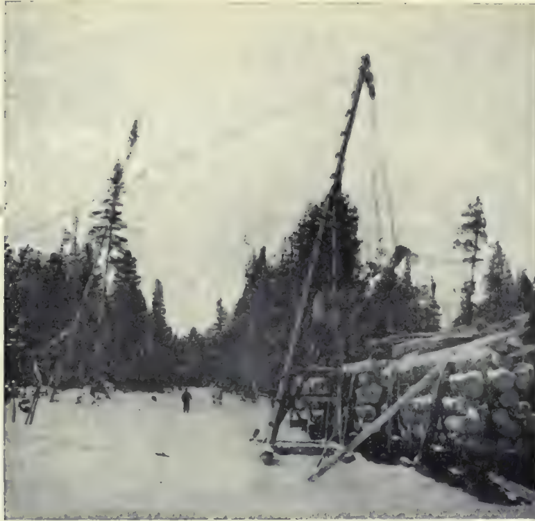
(1). PORTABLE GIN POLE ON SNOW SLED Sleigh on right being loaded from pile of logs (not shown) ; rope being pulled by horse.—River Marnie, Quebec.
