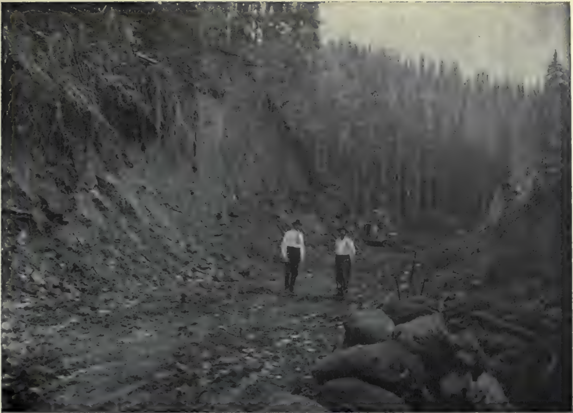
(1). Excavation of railway track by Marion Steam Shovel.—Elk River, Idaho.
