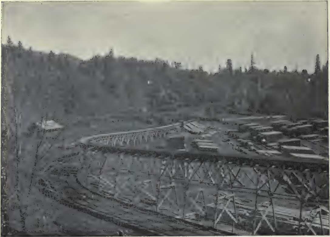
(1). Lower end of a flume bringing sawn timber from Mill to railway.—Lamoine, California.
