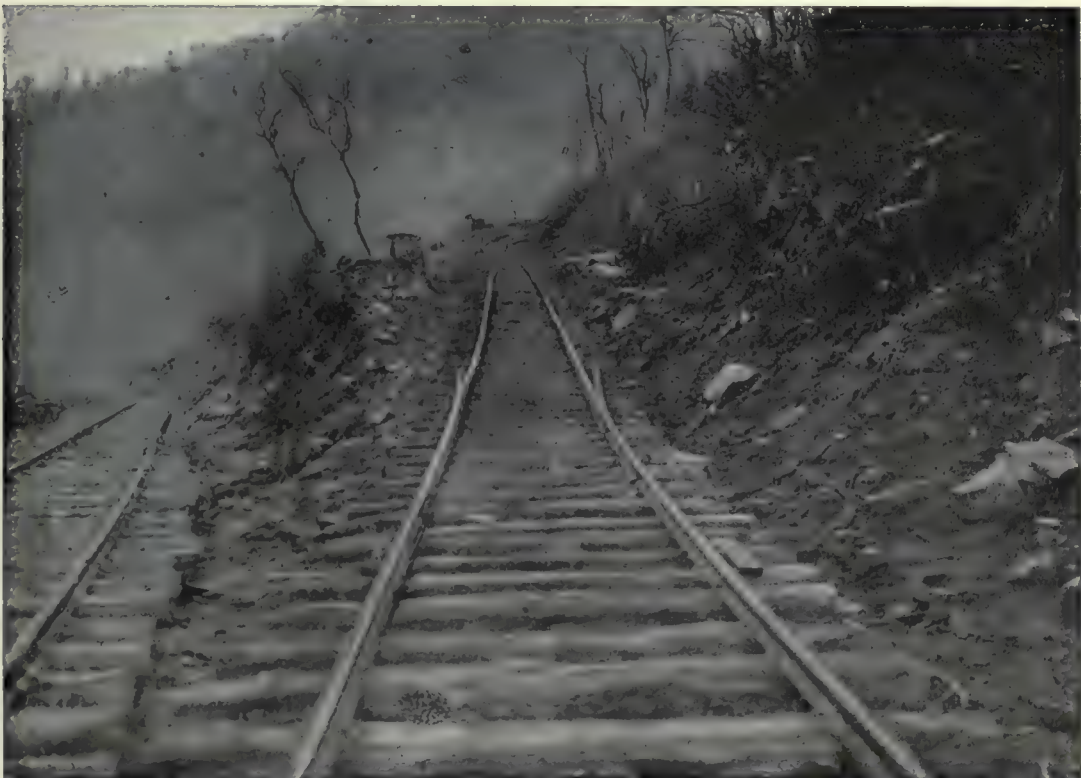
(2). Slip-Joints on log grades.—Townsend, Tennessee.
