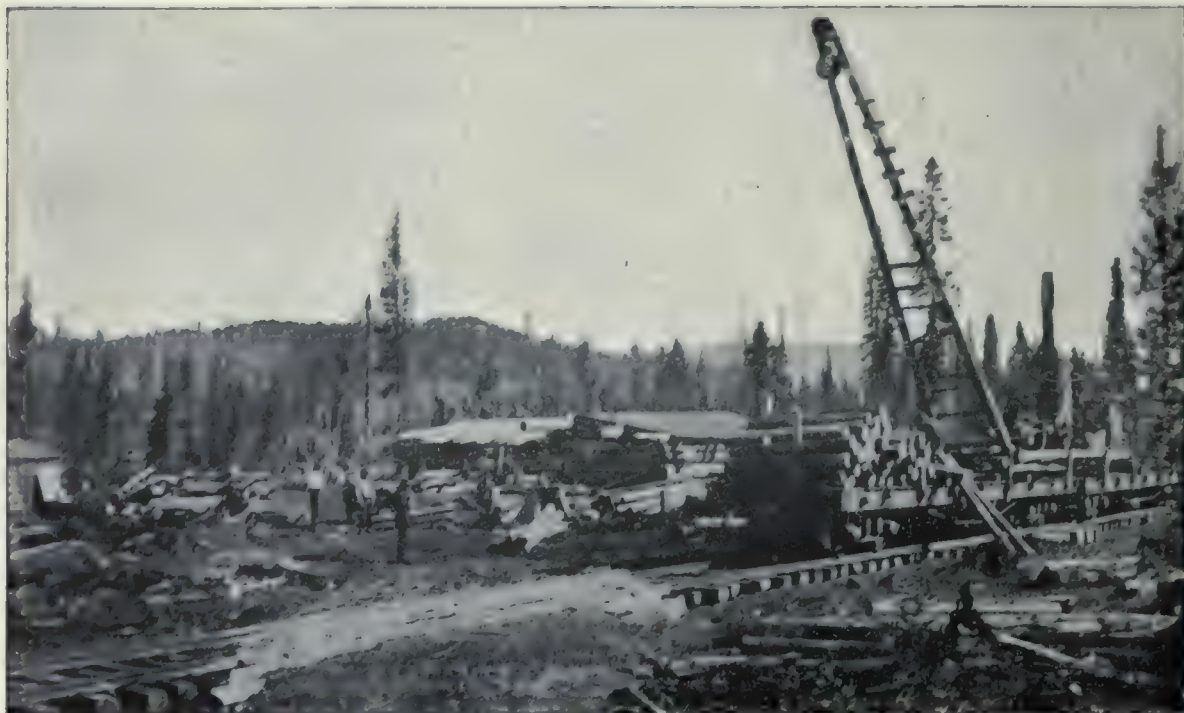
(1). Boom Skidder mounted on a railway car loading sleepers ;—Tyson Creek, Idaho.
