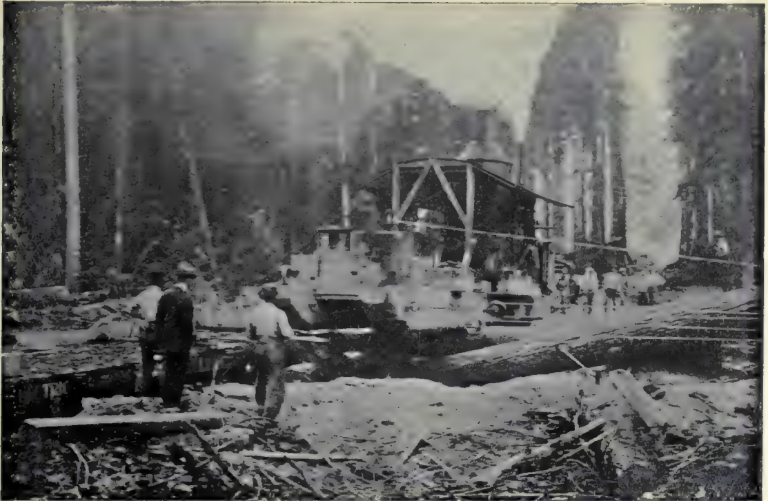
(1). Skidder mounted on timber skids hauling itself sideways off a railway car at a new setting ; New Westminster, B. C.
