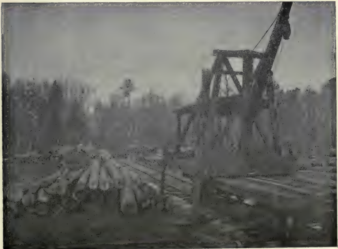
(2). Surry Parker Loader, empty car passing through :—New Bern, North Carolina.
