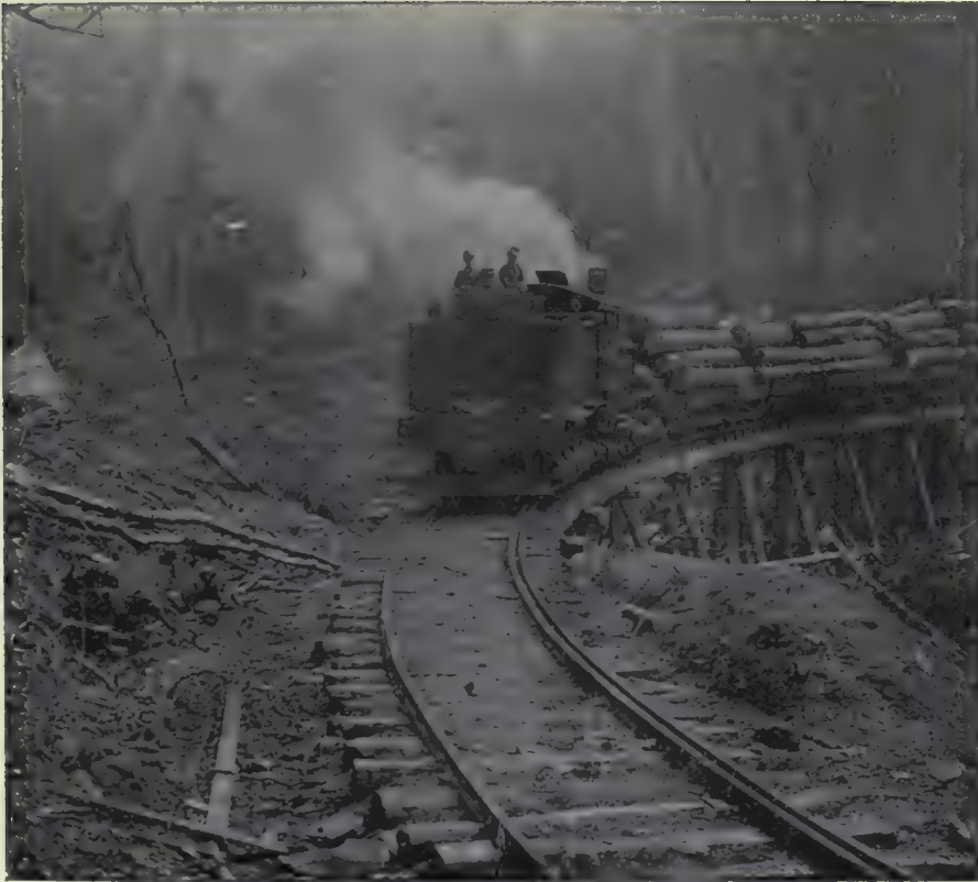
(1). Trestle and log train.—Townsend, Tennessee.
