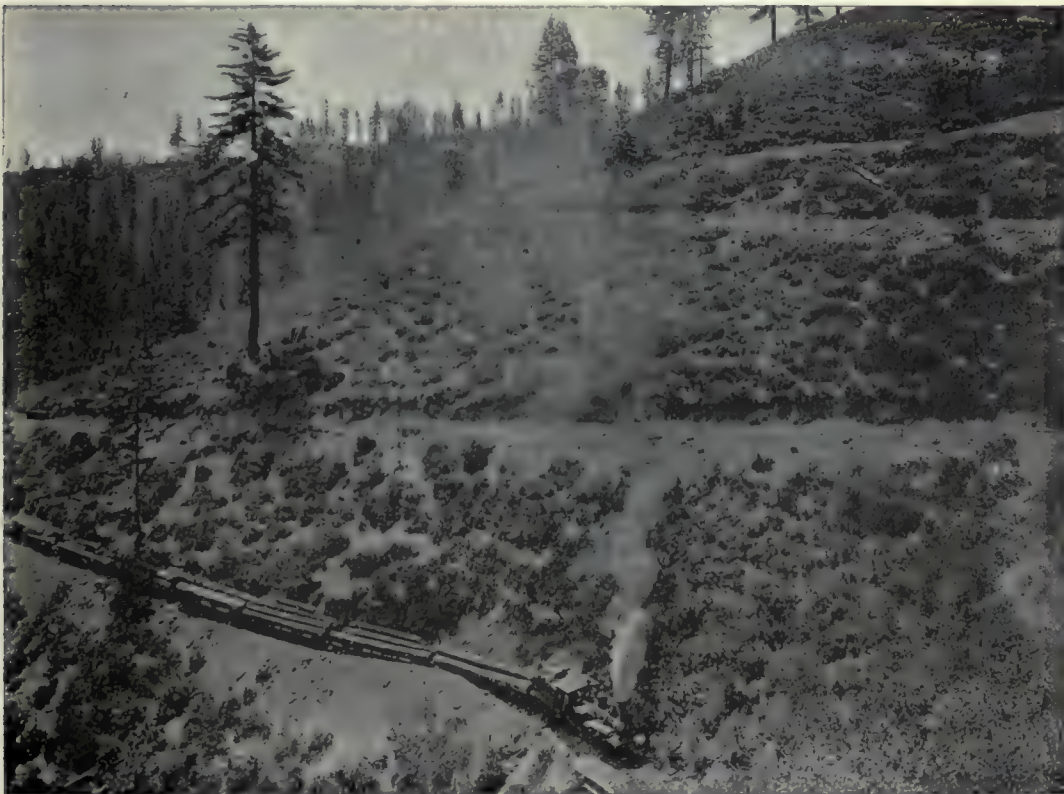
(2). Switch-backs and log train on 3-ft. track, Lamoine, California.
