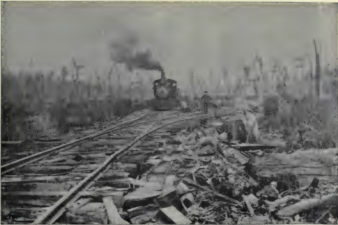
(1). Railway track in Cypress Swamp, showing ballasting with mill refuse.—Lutcher, Louisiana.
