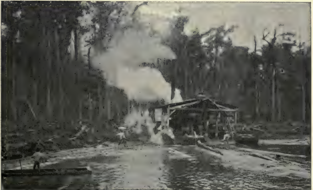
(2). Pull-boat at work in Cypress Swamp.—Donner, Louisiana.
