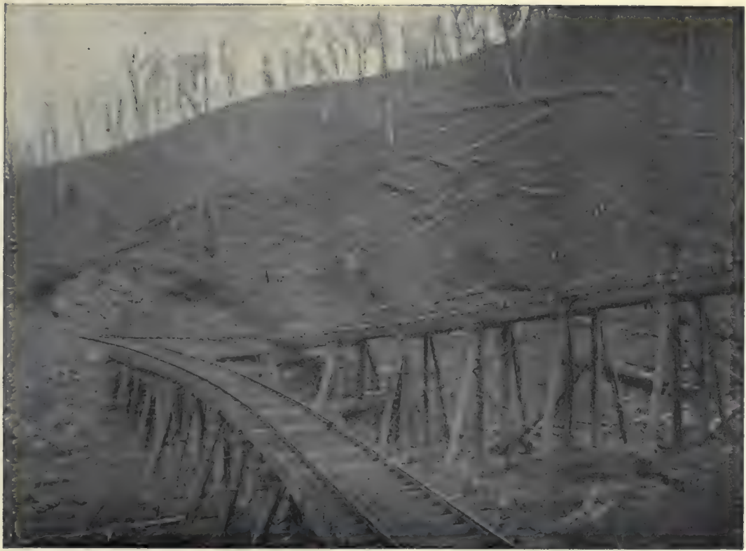
(1). Switch-back and trestles,—Townsend, Tennessee.
