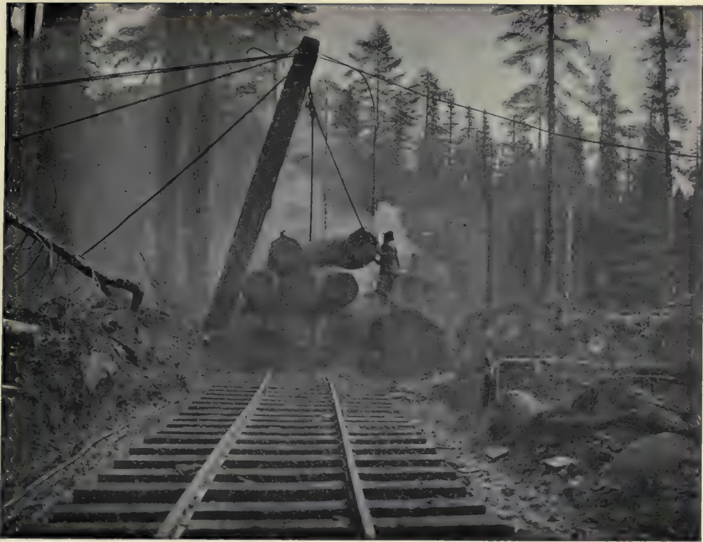
(1). Parbuckling by Steam Power ; 3 feet track.—Bridal Veil, Oregon.
