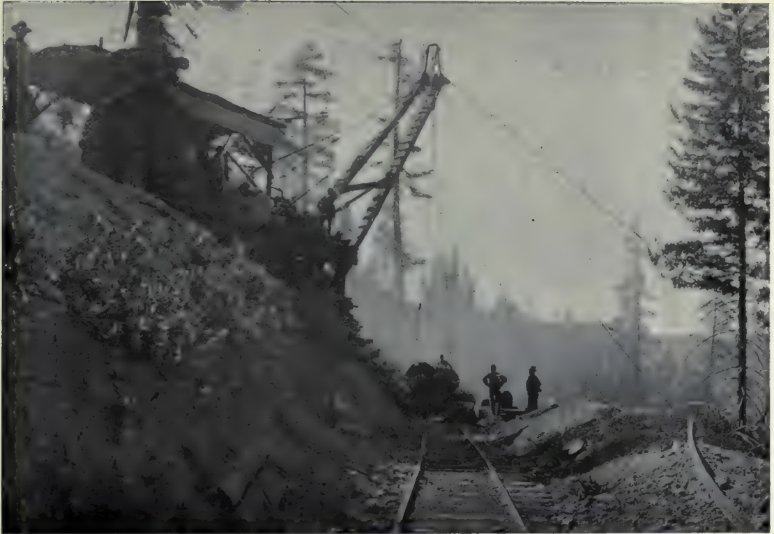
(1). Willamette Boom Skidder and Loader ; 3 feet track ;—Lamoine, California.
