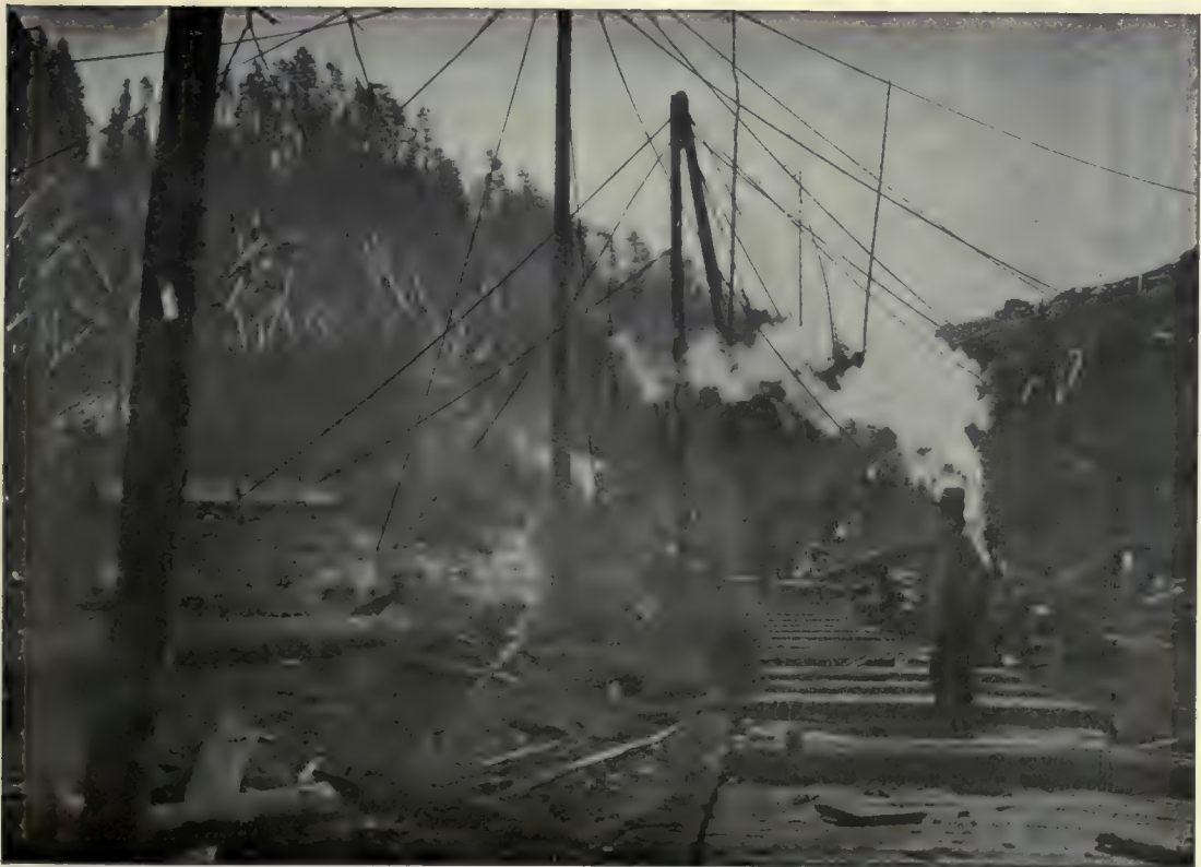
(2). Two-legged Gin Pole, 80 feet long.—Elk, California.
