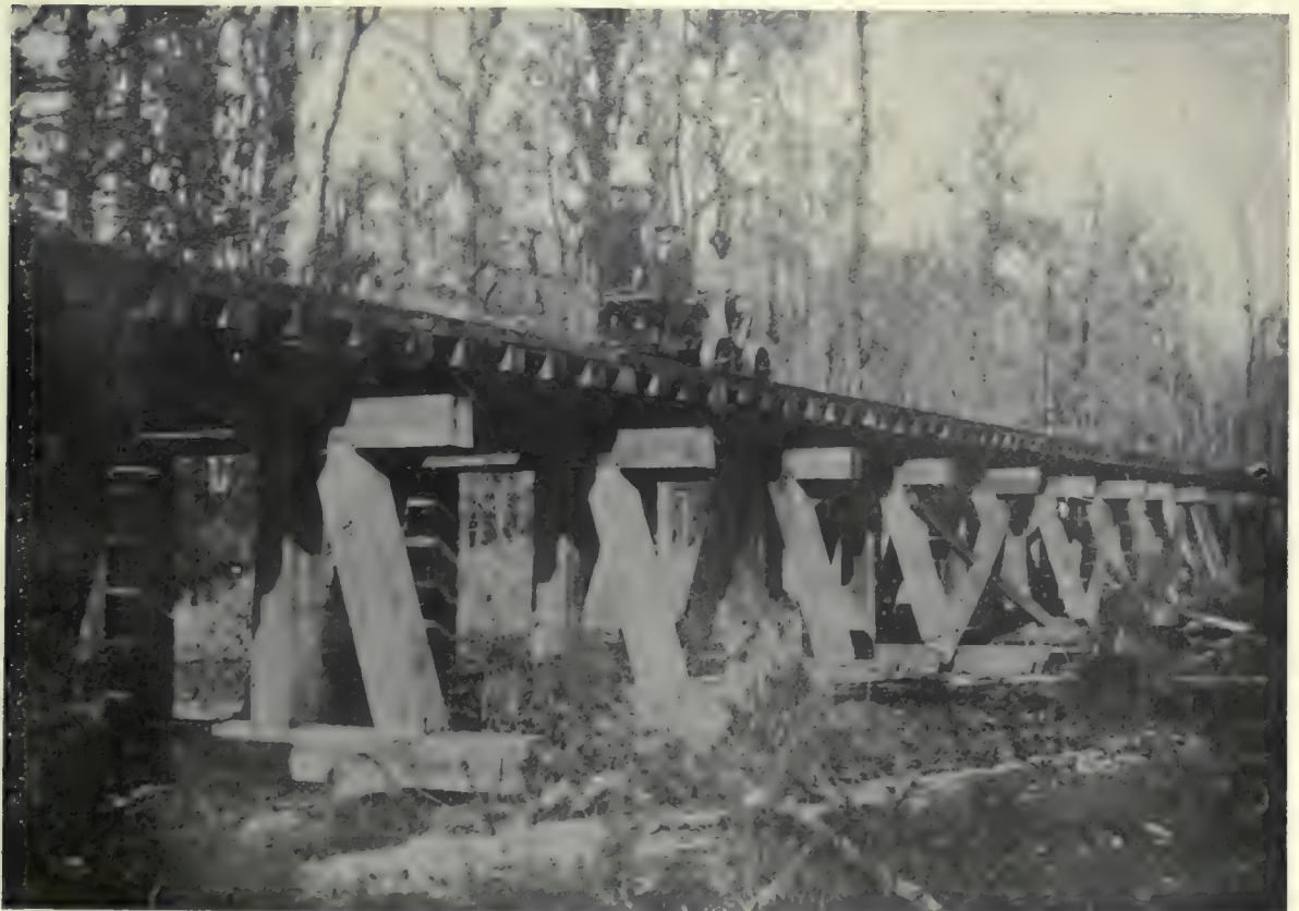
(2). Trestle across swamp,-New Bern, North Carolina.
