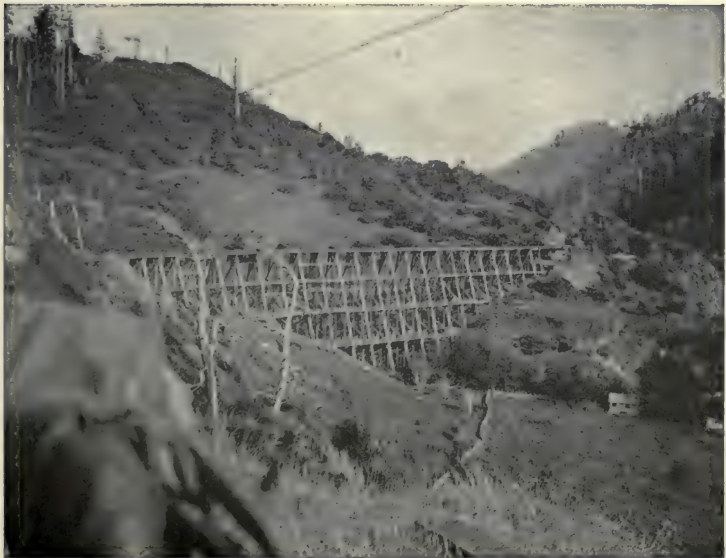
(2). Trestle 240 feet long and 150 feet high, 3 feet track.—Elk, California.
