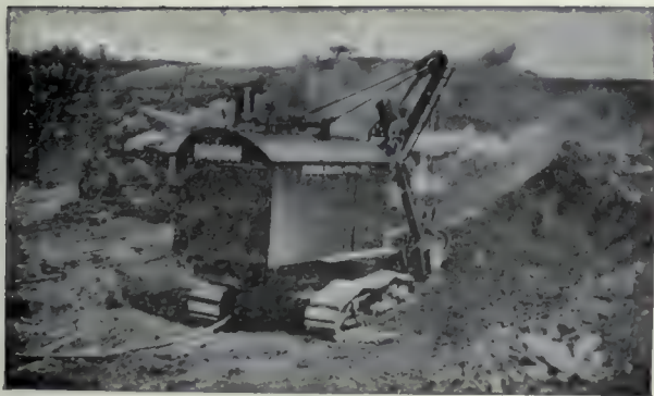
(2). Shovel mounted on caterpillar wheels.
