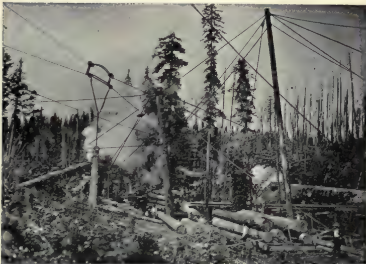
(2). Same as above at railway end of operation ; the smaller of the two spars is used for loading.—Keeler, Idaho.
