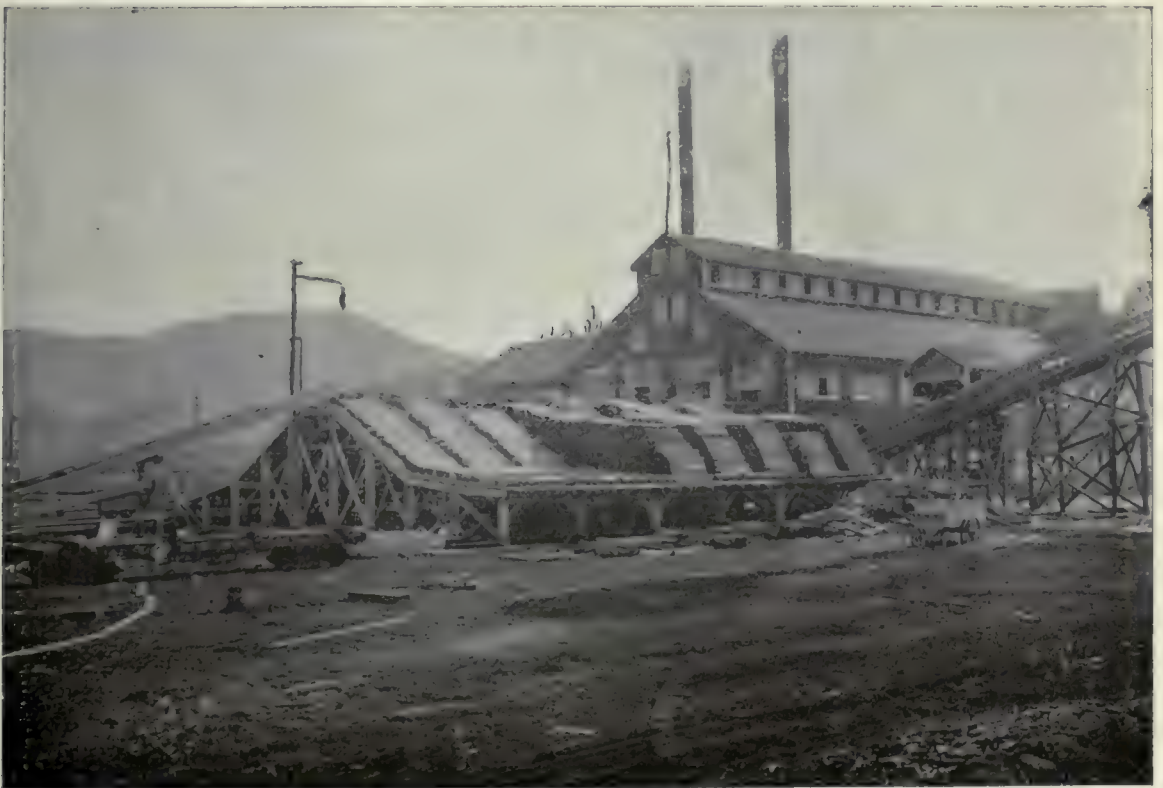
(2). Sorting and Loading Deck for sleeper.—Elk River, Idaho.
