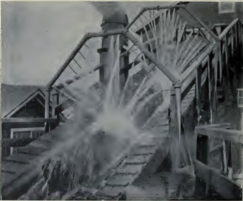
(1). Spraying of logs before entering mill,—Elk River, Idaho.
