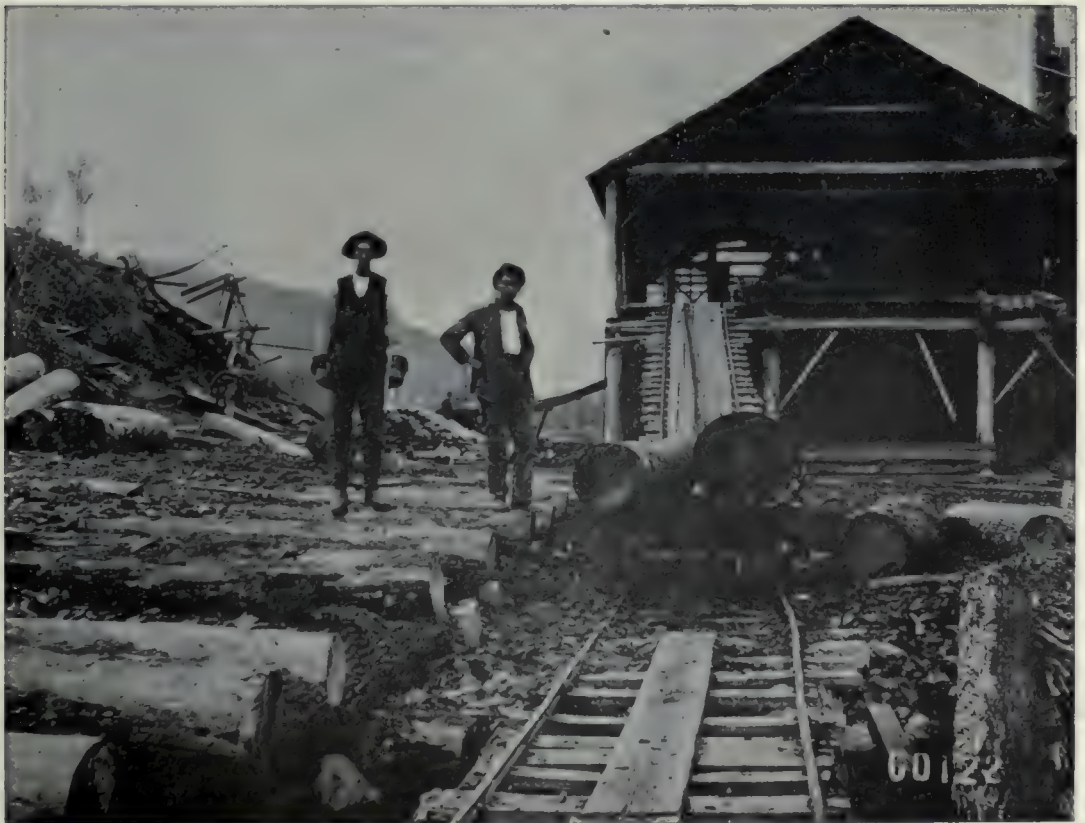
(2). Trolley and Cable method of hauling logs in to a mill.
