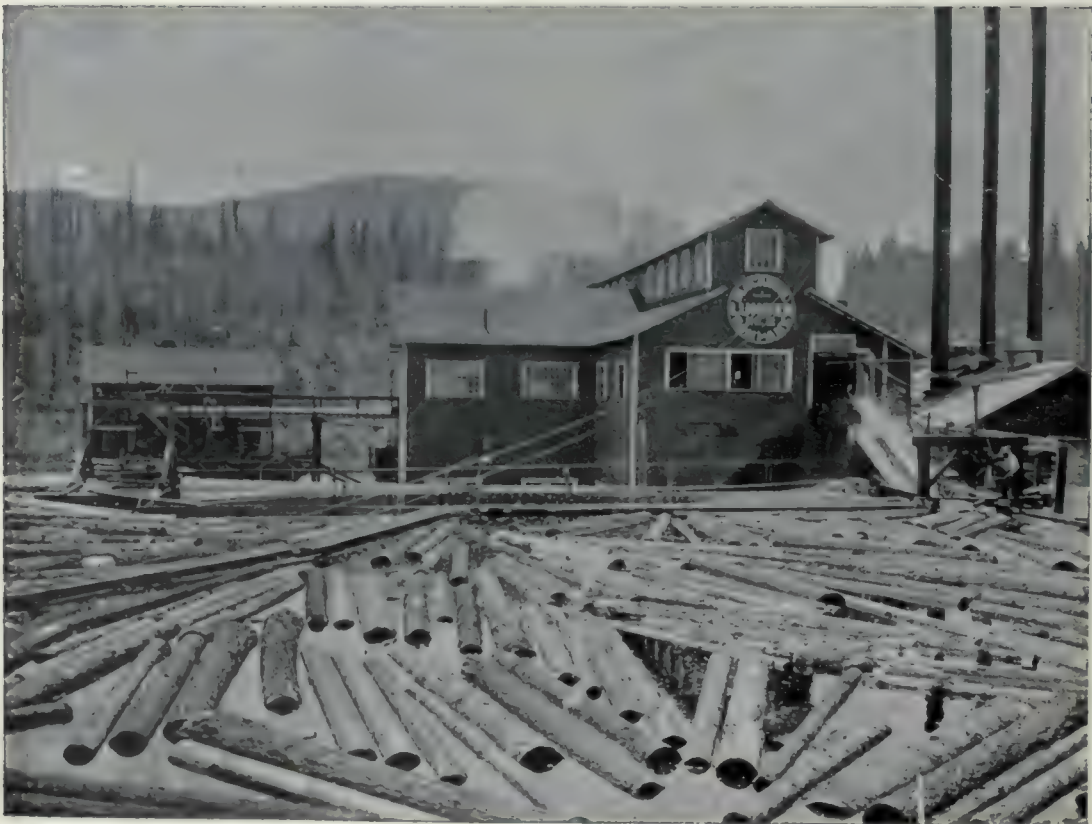
(2). Mill Pond and spraying of logs ;— Fernwood, Idaho.
