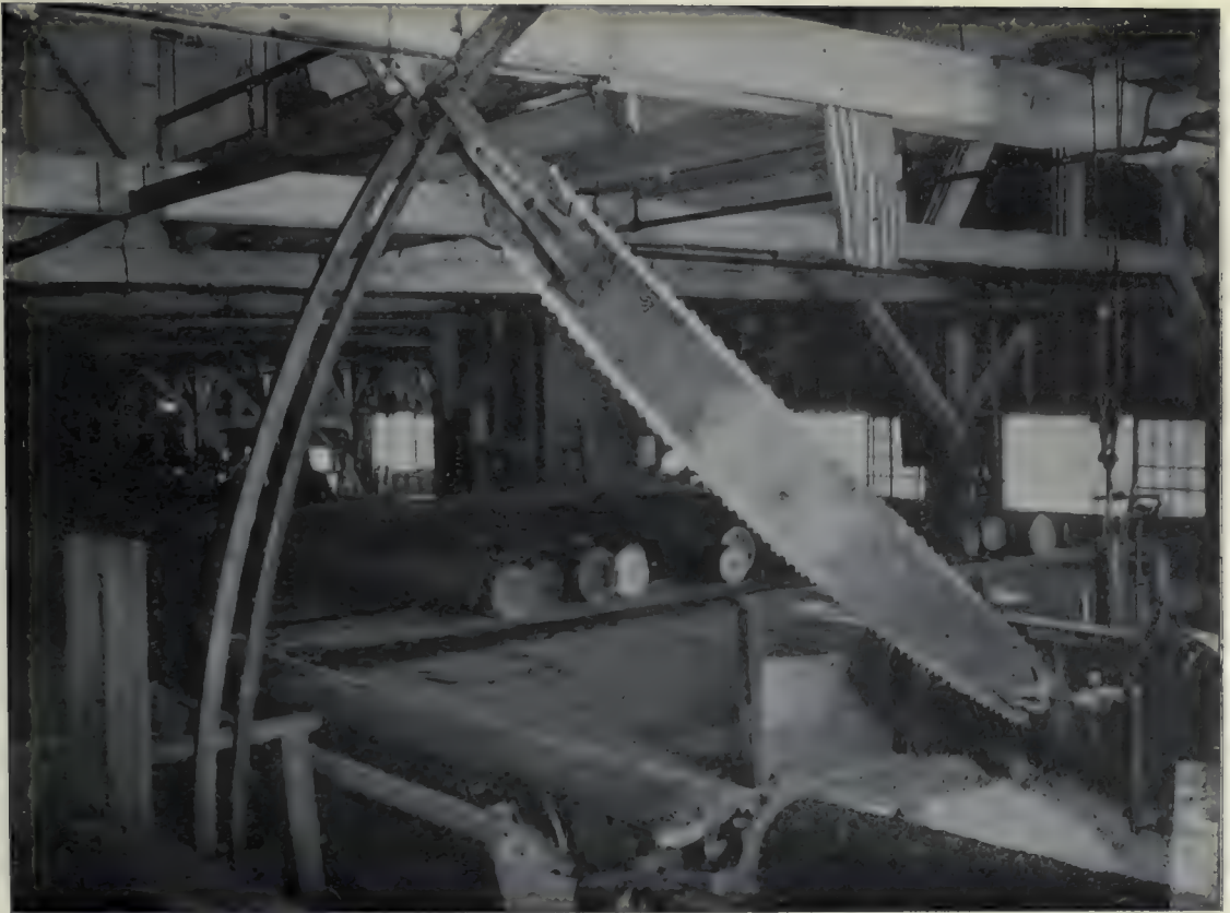
(1). Chain saw for cross-cutting inside mill—Elk River, Idaho.
