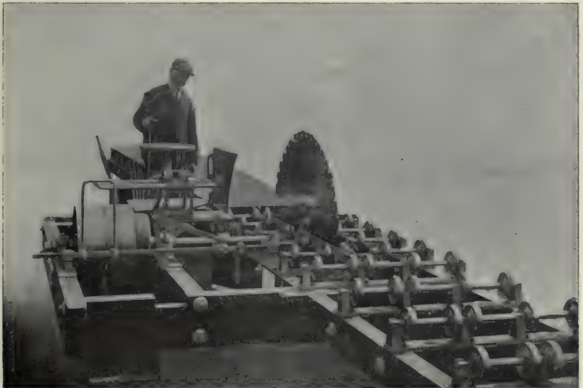
(2). Plain Rack Feed Log Table of British design with 3 speeds operated by separate levers. (By permission of Messrs. Stenner and Gunn). In both of the above designs the feed is positive ; the speed cannot be varied by allowing the belt to slip.
