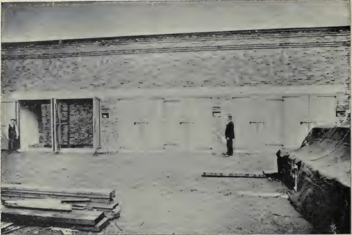
(1). Sturtevant Compartment Kilns, put up for the British Air Board. (Presented by Mr. Fitzgerald).
