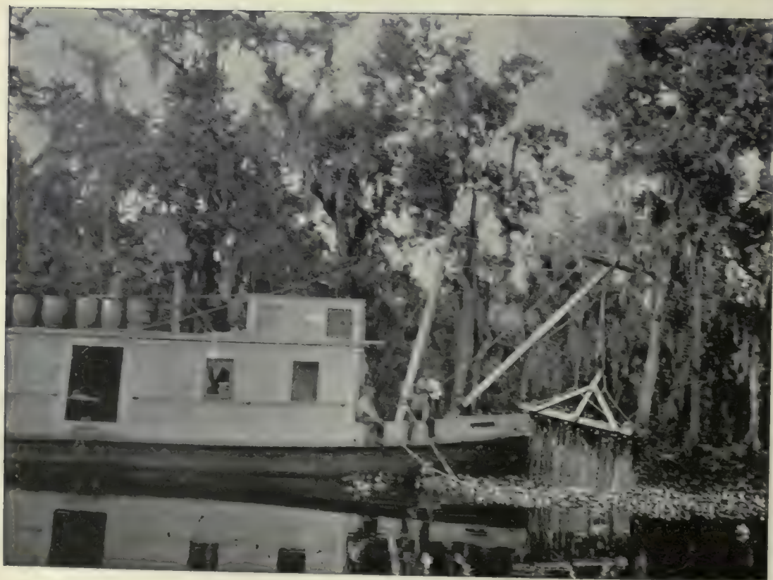
(2). Grappler at work, grapple being raised ;— Haw Creek, Crescent City, Florida.
