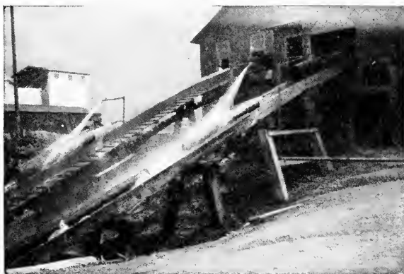
FIG. 17.—Log-washing Equipment installed on a Jack Ladder.
