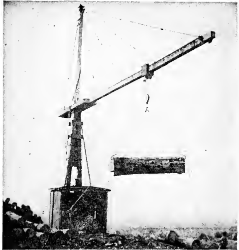
FIG. 6.—A Portable Log Unloader and Stacker for Hardwood Operations.
