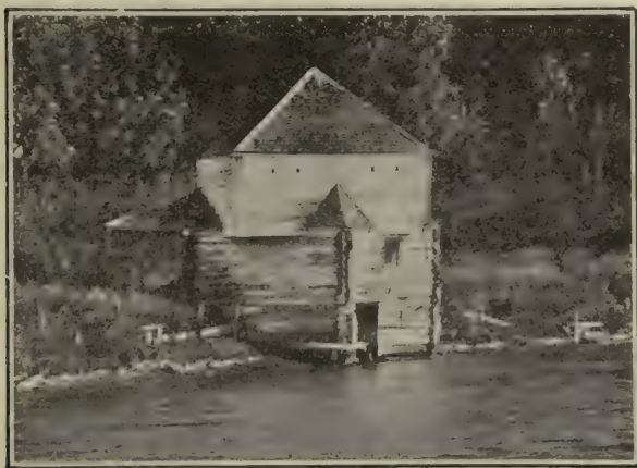
Old English Blockhouse on San Juan Island. Built in 1856. Roof of Western Red Cedar shingles still in good condition, after nearly 60 years' service without paint or repairs
