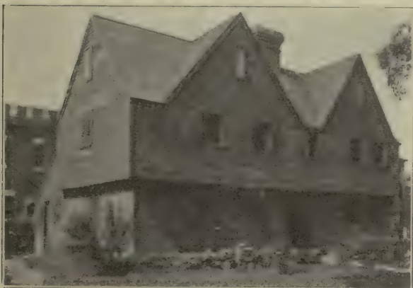
House at Salem, Mass., sided with White Pine in 1684, and well preserved after 230 years
