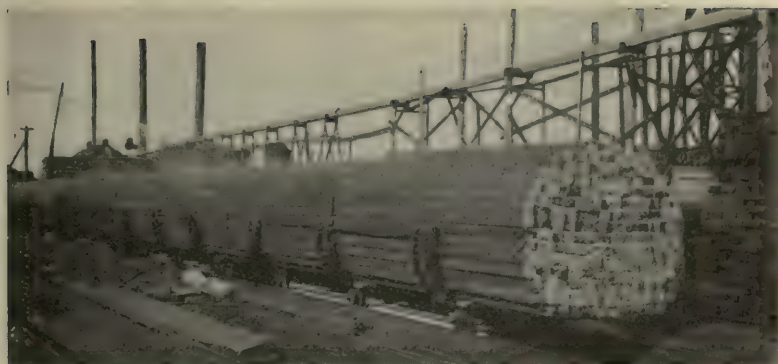
Creosoted Cross-Arms Shortly after Removal from Treating Cylinder
