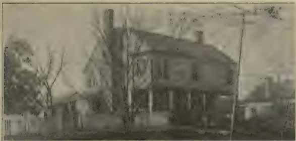
House 150 years old, built of Southern Yellow Pine throughout, including siding, and still in a state of good preservation
