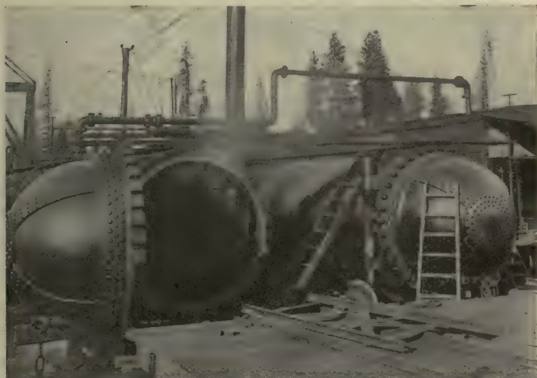
Portable Plant of Cylinder Type for Creosote Treatment of Railroad Ties
