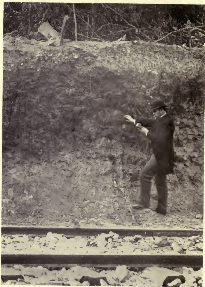
VIEW WEST OF CHEVY CHASE, MARYLAND
