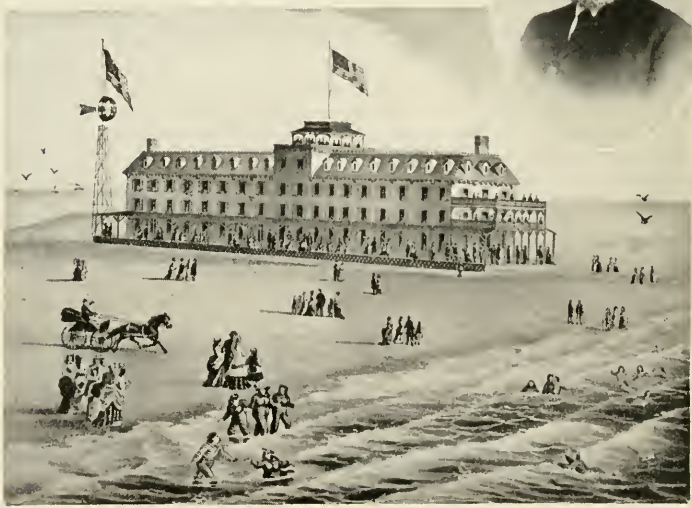
The Engleside The Parry House
