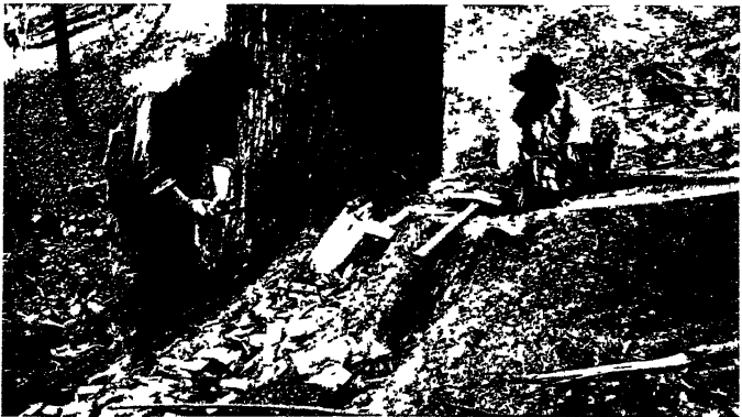
WORKING ON THE 'PUBLIC WORKS'
