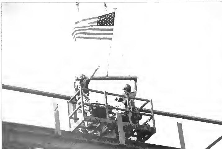
Larry Allison '96 (at left) helps to secure the last piece of structural steel on the Rec Center.
