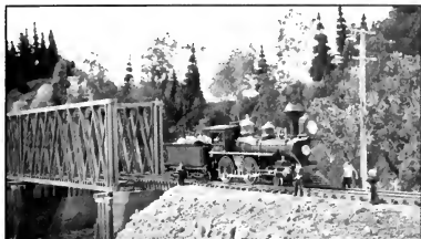
Model of an Oil Creek Railroad train stopping at the Pioneer, Pennsylvania, Railroad Bridge, circa 1866.
