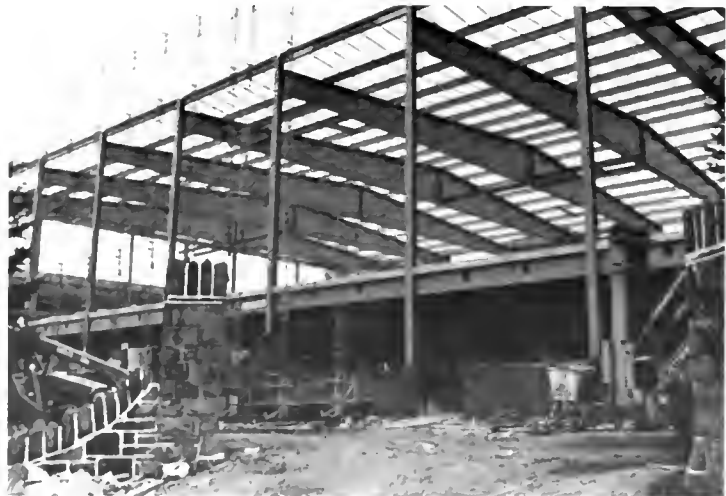
PHOTO BY W. W. The shiny, new steel girder of the new Physical Education and Recreation Center rise high above the ground level above the Lycoming College campus—the main gate to the old Williamsport, Pa. campus, Pennsylvania State College, where the workers carried into the site earlier at the left.
