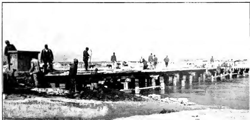
ITALIAN BRIDGE OVER THE CERNA AT BROD.
