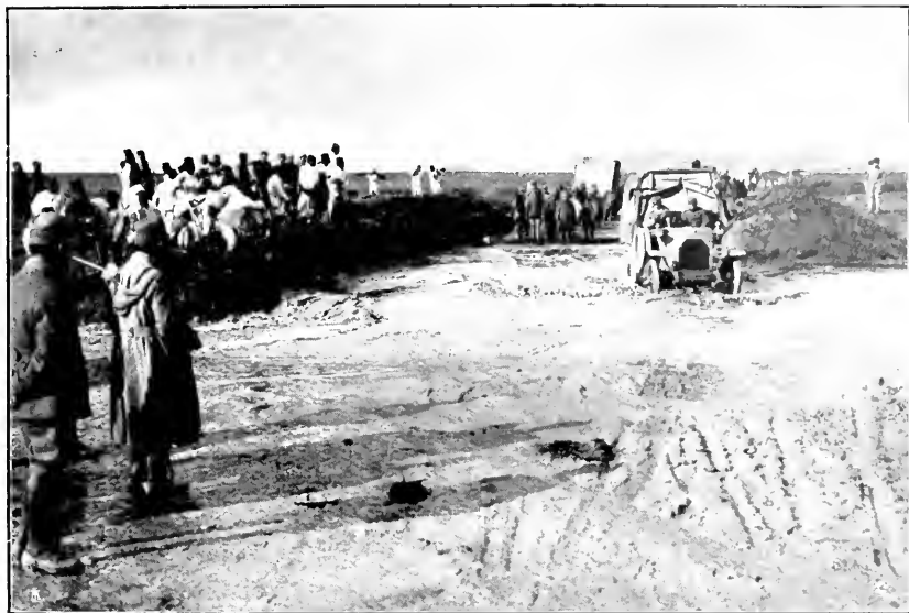
A FLOODED ROAD.
