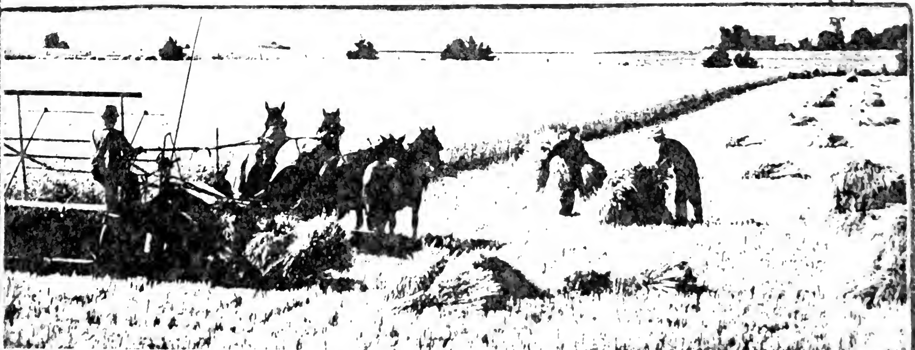
The binder, with its slow reel and canvas conveyor, was designed to handle grain gently to avoid threshing prematurely.
