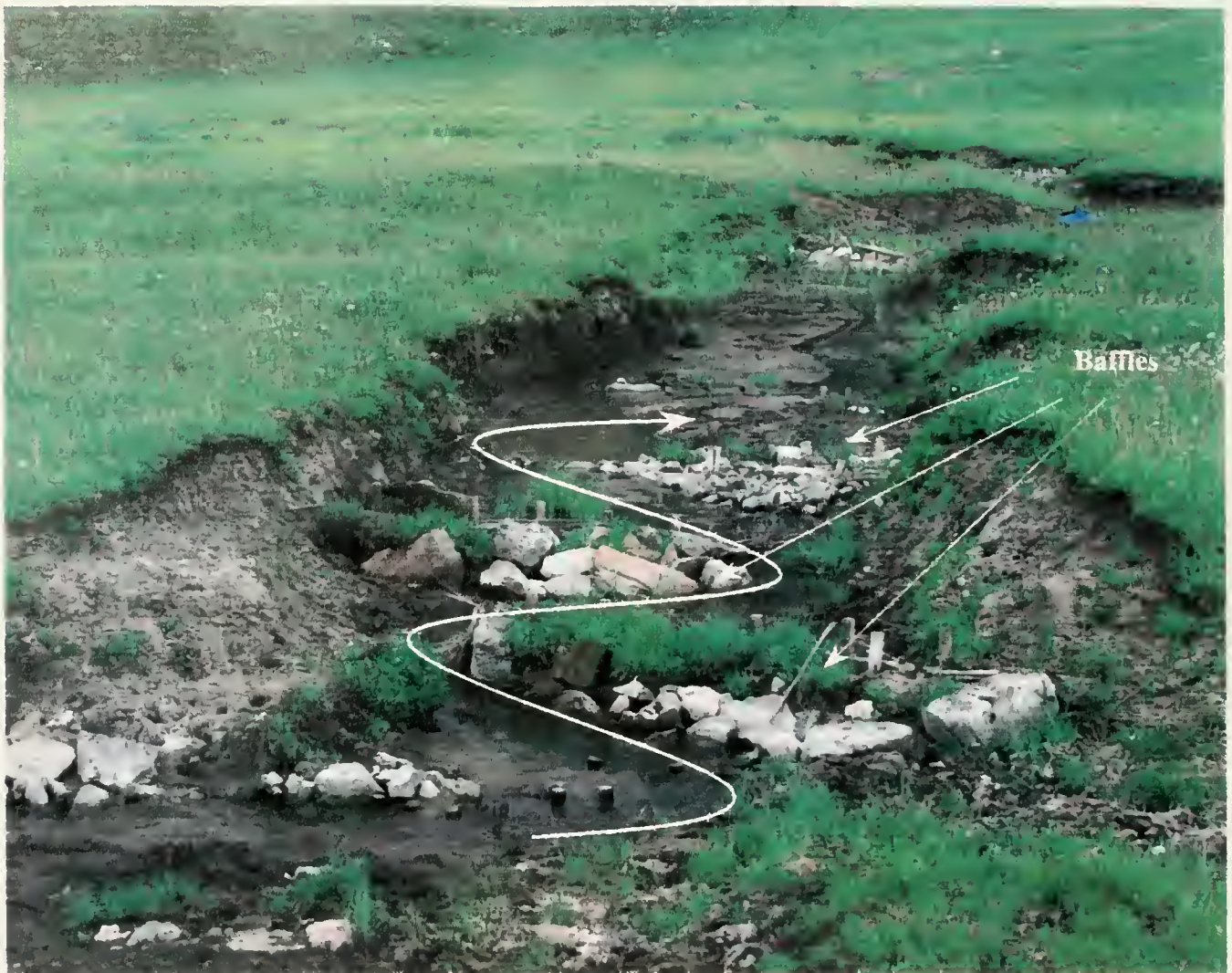
Figure 2. View looking downstream at a series of baffles built in 2006 that induced meandering, July 2007.
