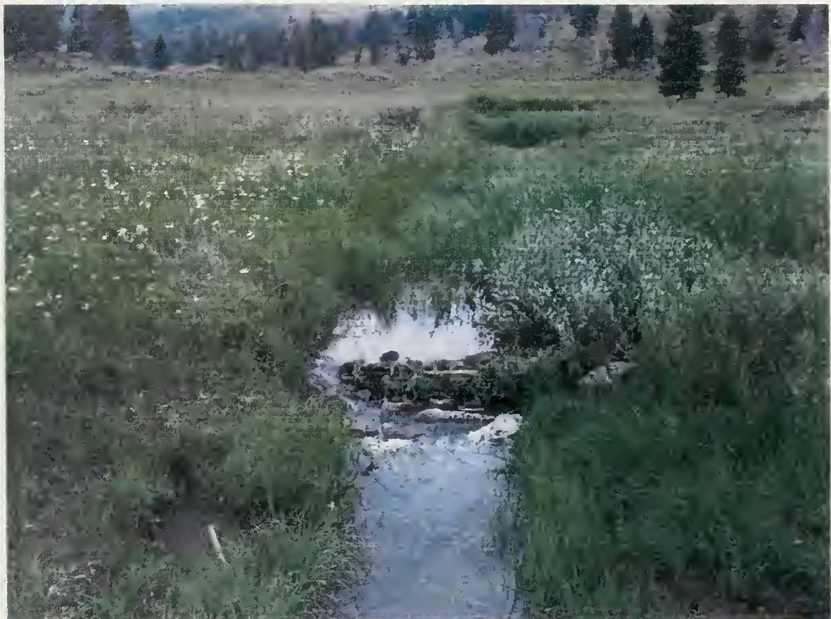
Figure 4. Riffle with fish passage at left, raising water surface elevation about 2 feet. 2007.
