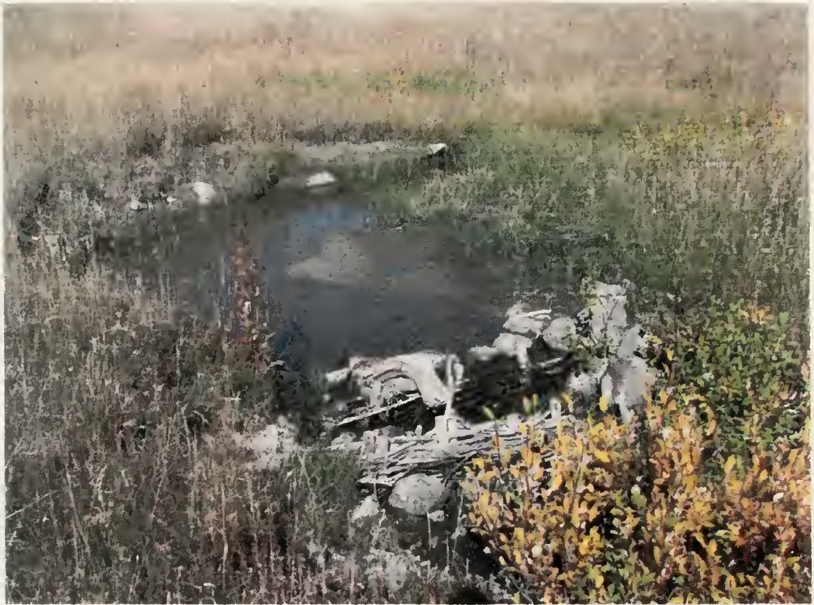
Figure 3. Same structure following long duration spring runoff, July 2008.
