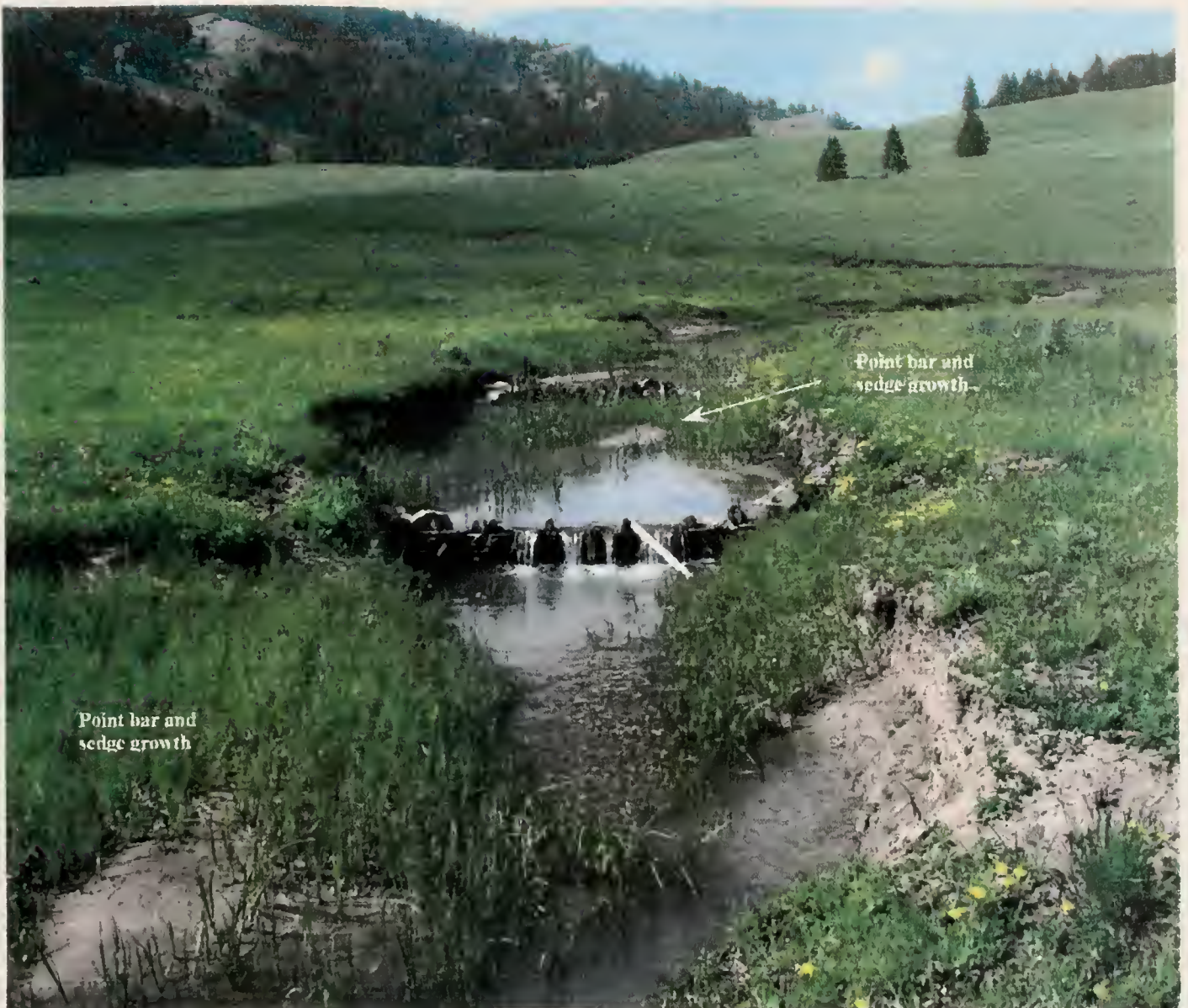
Figure 7. A weir trapping large amounts of sediment and raising the surface water level, July 2008. Sedge recruitment is already occurring on the point bars, and spawning gravel has been sorted in the thalweg below the weir.
