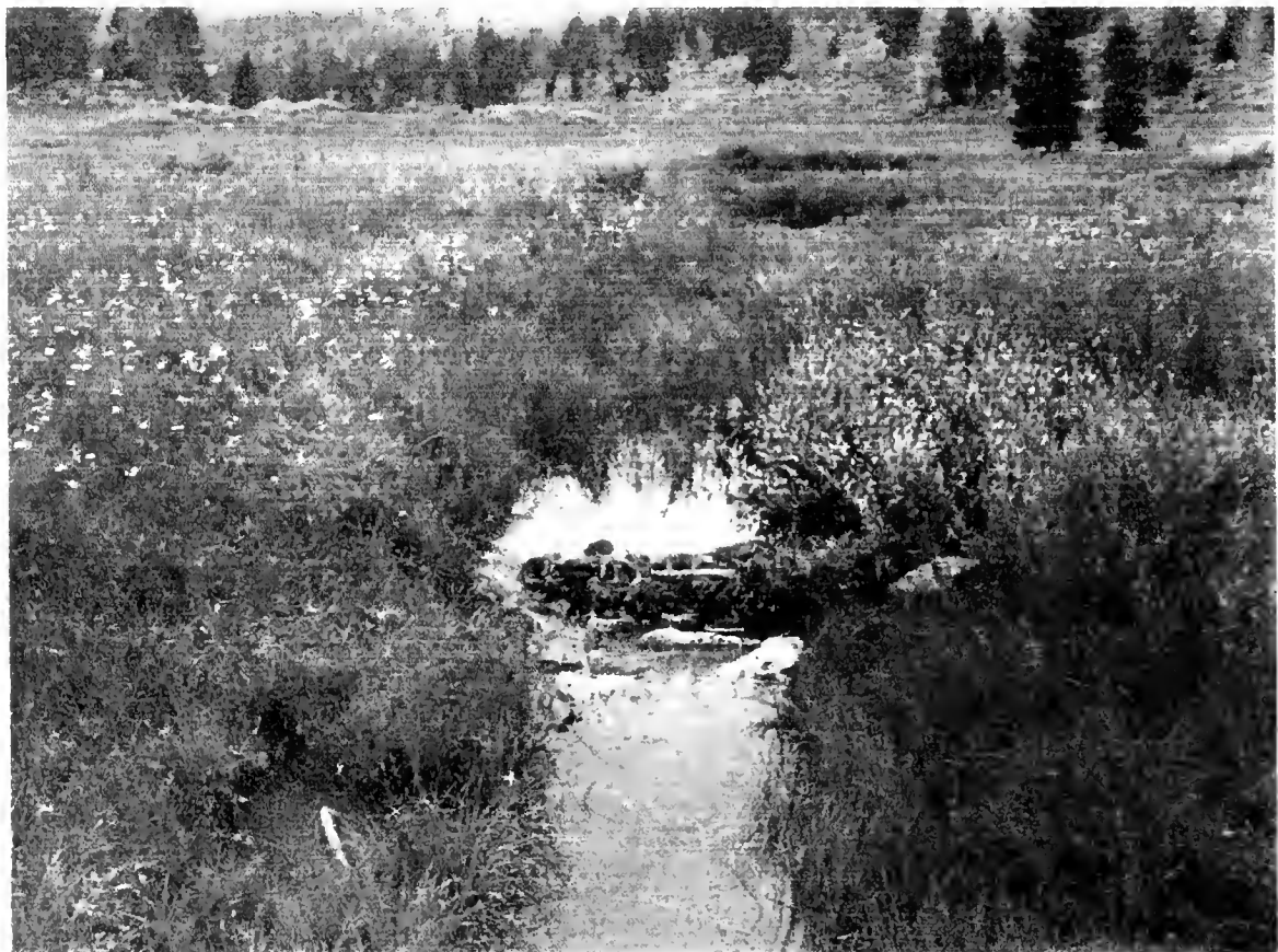
Figure 4. Riffle with fish passage at left, raising water surface elevation about 2 feet. 2007.
