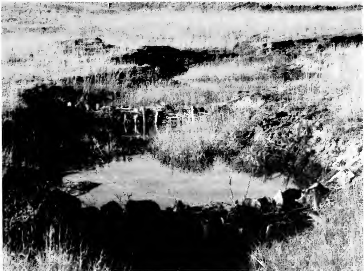
Figure 1. Channel spanning weirs composed of wood stakes, willow, rock, and sedge plugs, September 2006.
