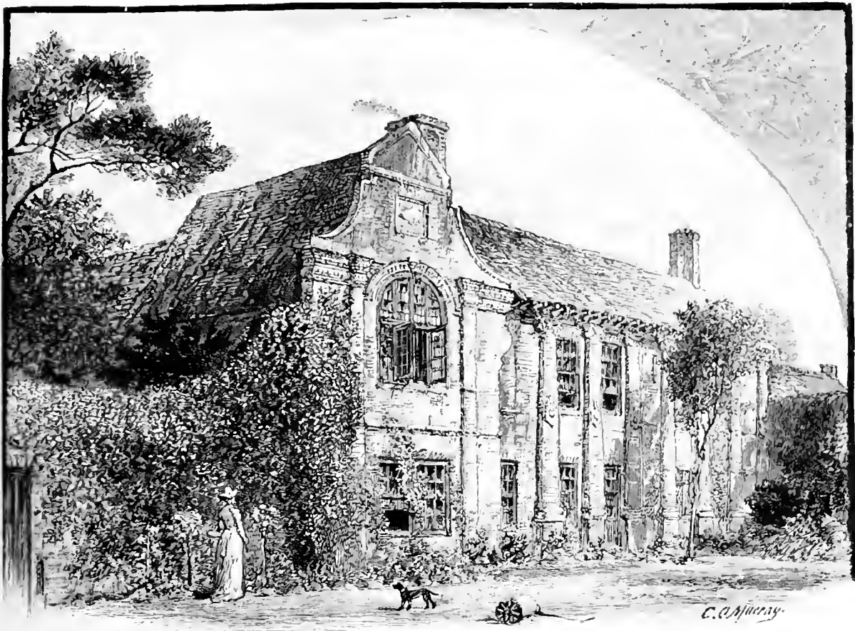
1.—SLYFIELD HOUSE: THE GARDEN FRONT.
