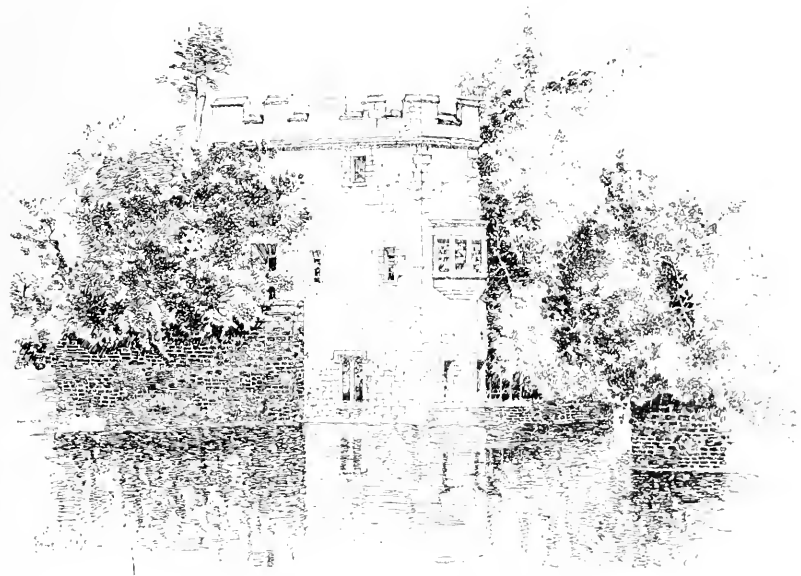
GATE-HOUSE AND MOAT TO THE BISHOP'S PALACE, WELLS.
