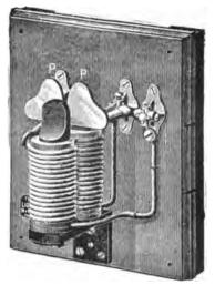
FIG. 64.—ELECTROMAGNETIC LIGHTNING ARRESTER. ful magnetic flux upon a voltaic arc is to push it aside or violently distort it. The electromagnet, therefore, acts as an extinguisher of the electric arc, and, in the
