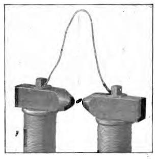
FIG. 71.—DIAMAGNETIC SUBSTANCE BETWEEN MAGNET Poles.
