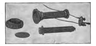
FIG. 56.—PARTS OF AN ORDINARY BELL TELEPHONE.
