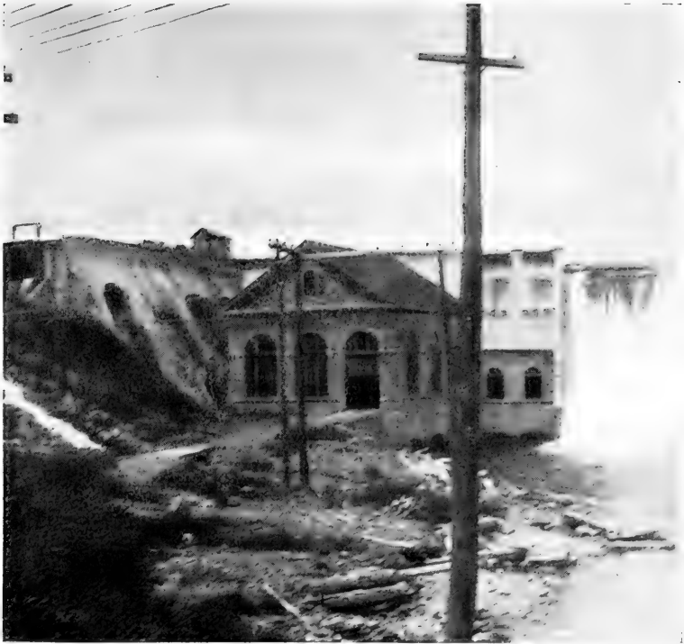
Power Plant at Ellsworth
