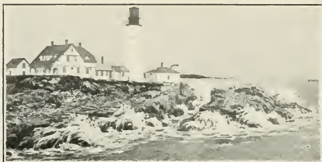
PORTLAND HEADLIGHT, PORTLAND HARBOR
