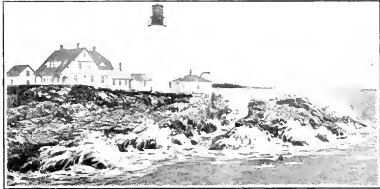
PORTLAND HEADLIGHT, PORTLAND HARBOR
