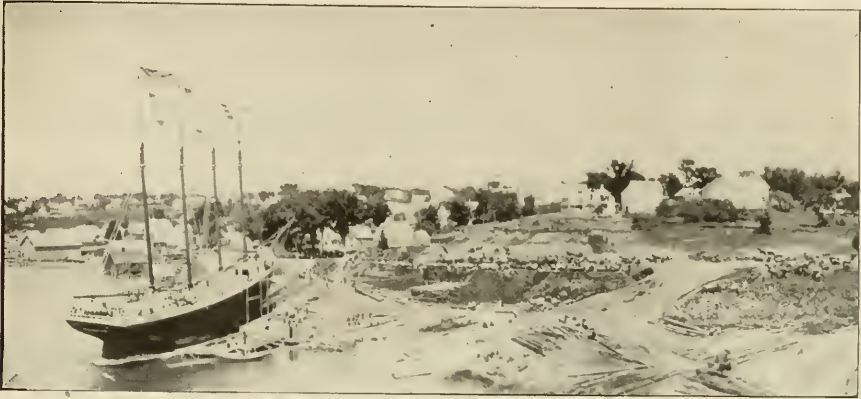
LAUNCHING OF THE L. HERBERT TAFT AT THOMASTON
