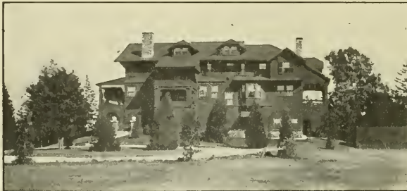
SNEATH COTTAGE, BUILT BY S. G. RITTERBUSH
