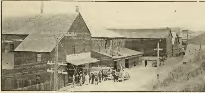
FRONT VIEW OF CAMDEN LUMBER CO.
